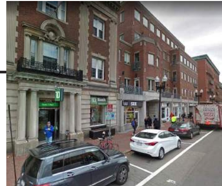
Existing metalwork details on Massachusetts Avenue
