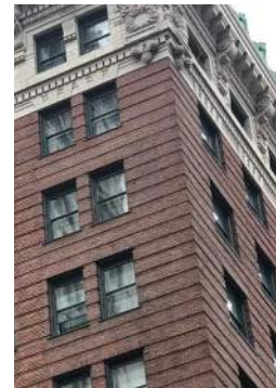
Detail in Brick
