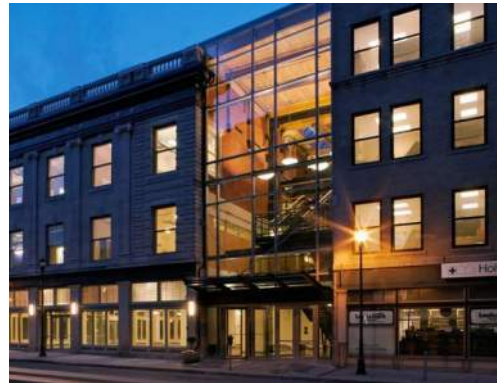
Existing masonry wall is featured through the glazing
