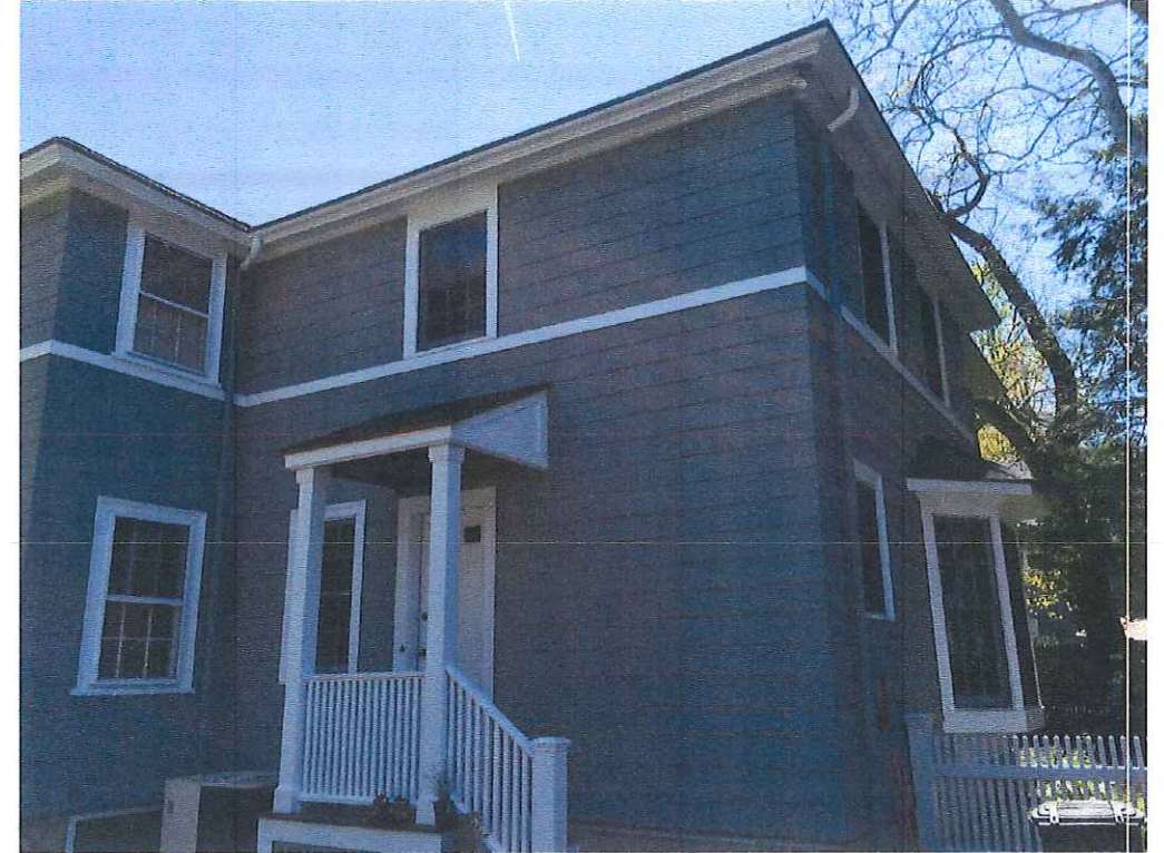
EXISTING BAY AND SECOND FLOOR WINDOWS
