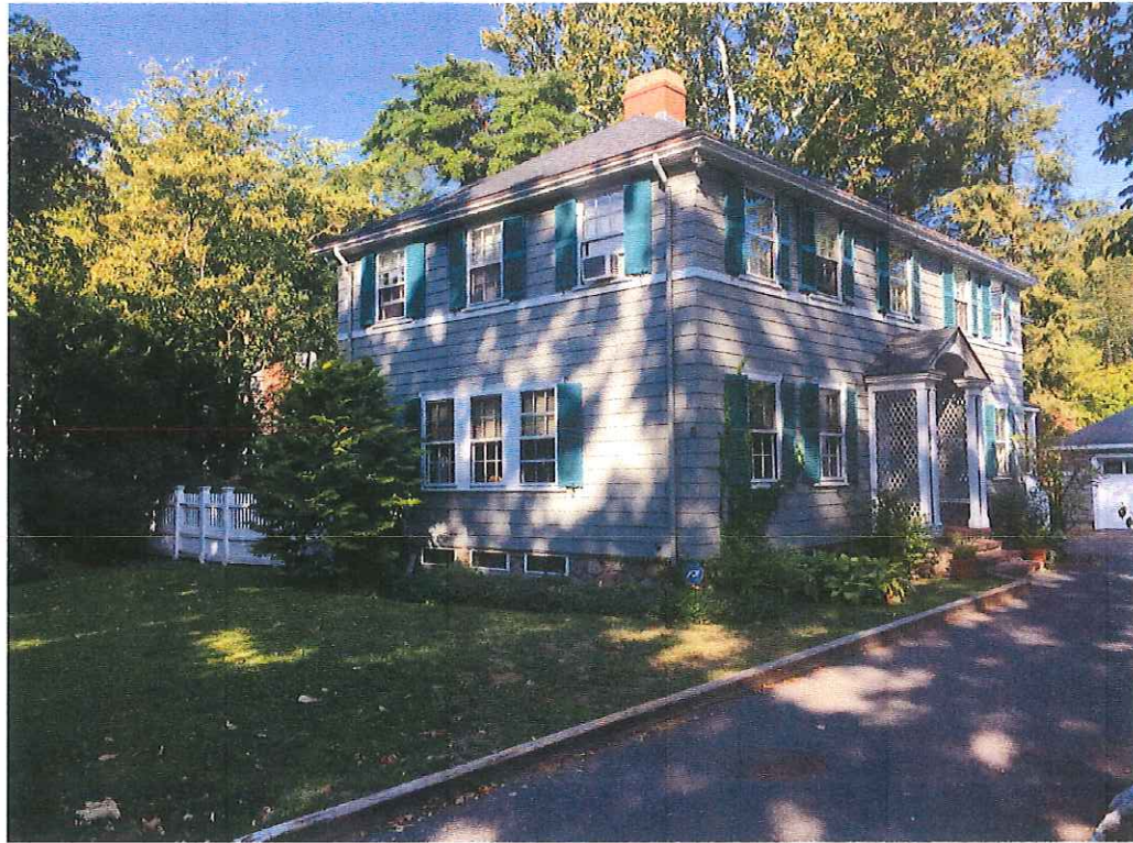
PROPERTY LOOKING WEST FROM BERKELEY PLACE
