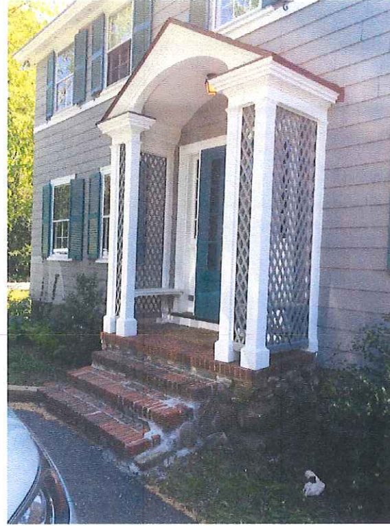
FRONT STEPS AND LANDING
