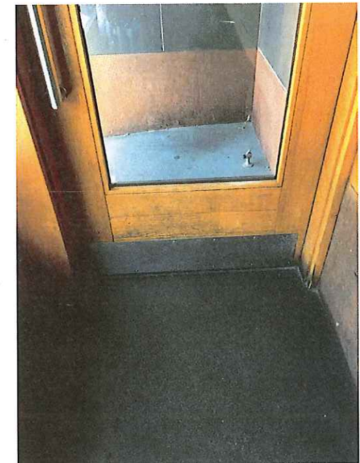
EXISTING CONDITIONS OF PROPOSED SECONDARY EXIT
