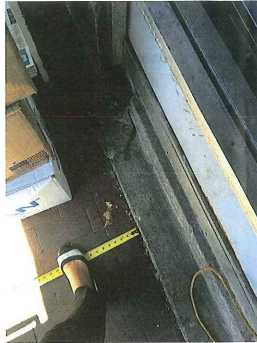
CLOSE UP OF BRICK AND CURB CONDITIONS
