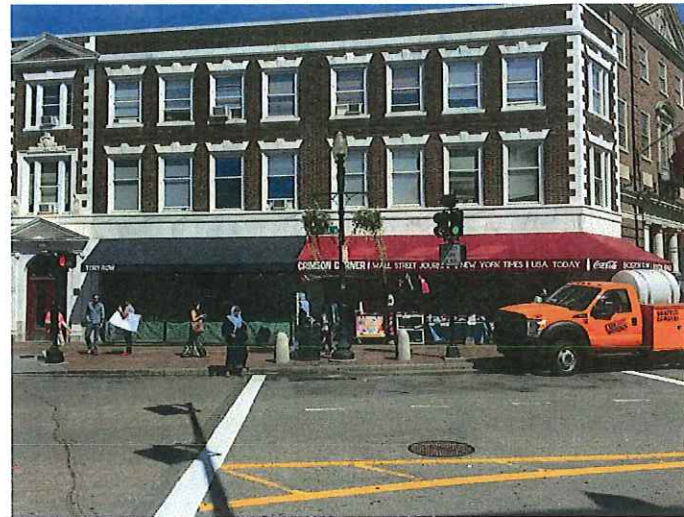
EXTERIOR FACADE AND STREET CONDITIONS. BIRCK AND MARBLE TO REMAIN AS IS
