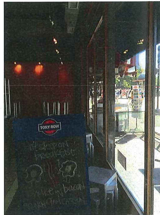
INTERIOR VIEW OF EXISTING TORY ROW FACADE
