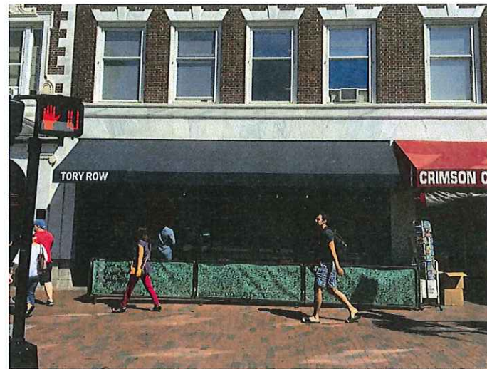
EXISTING TORY ROW FACADE AND PATIO CONDITIONS
