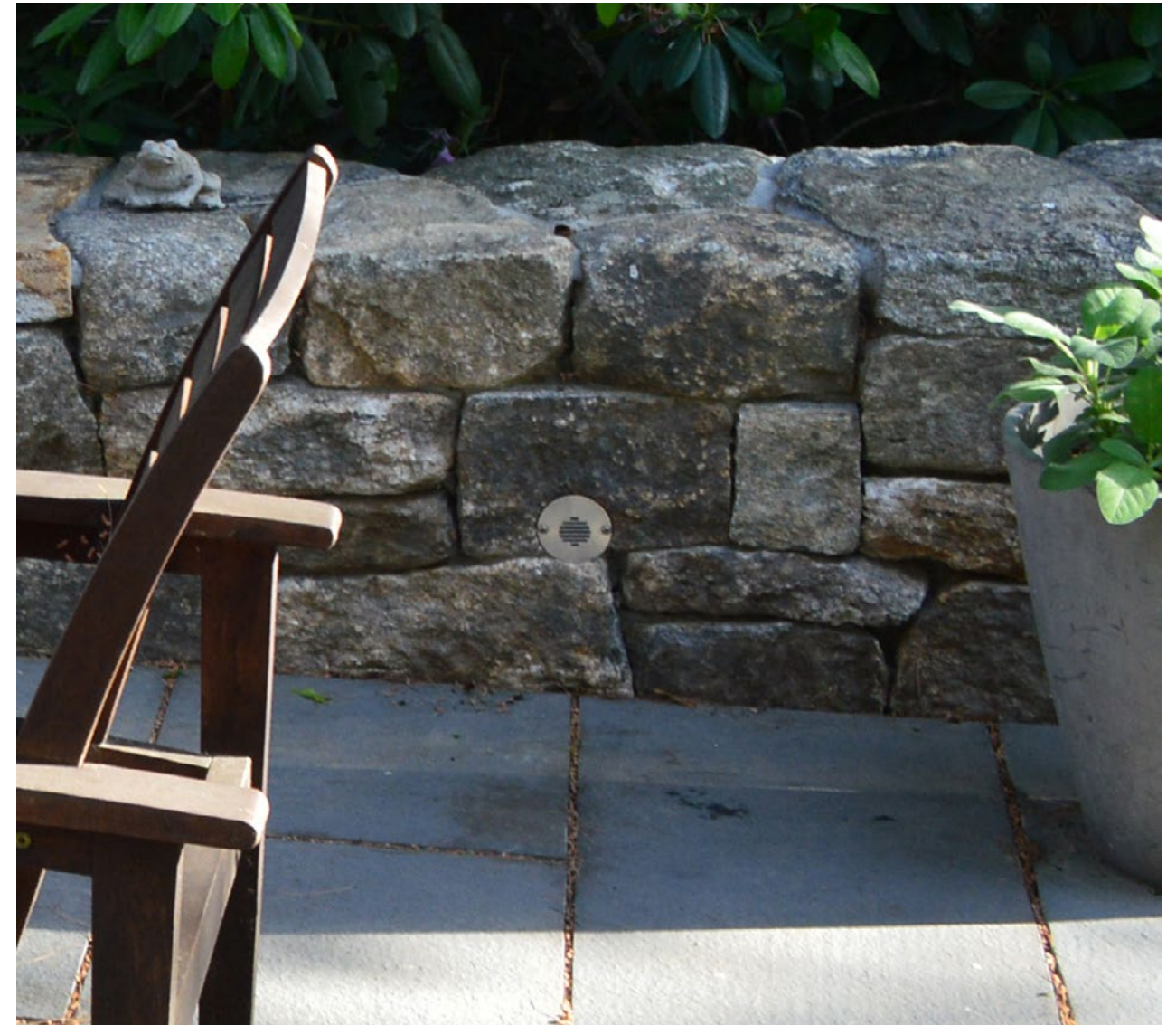
Flush louvered light in face of benches ( 2 per bench)
