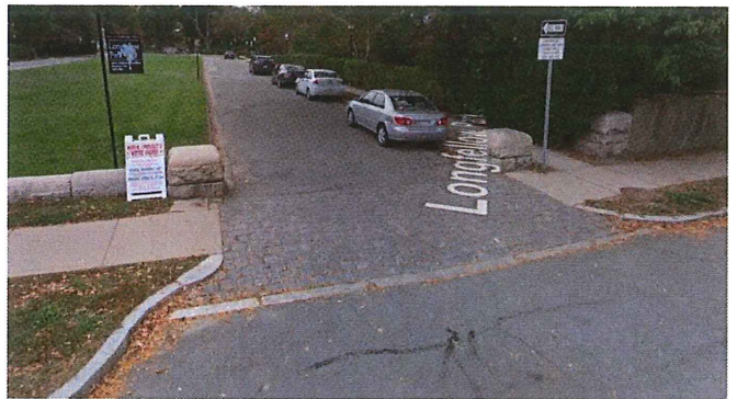
Existing non-accessible granite pavers - Longfellow Park (west)
