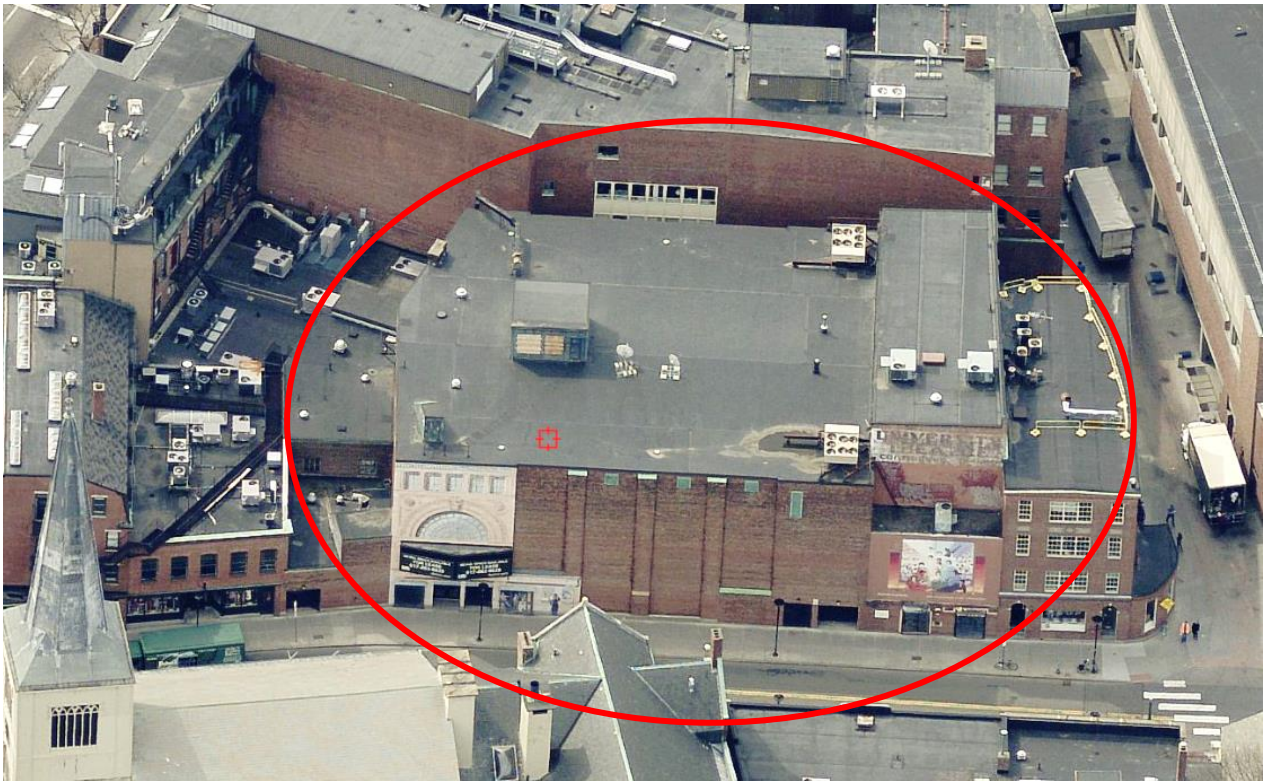
10 Church Street, northerly view, 2014
