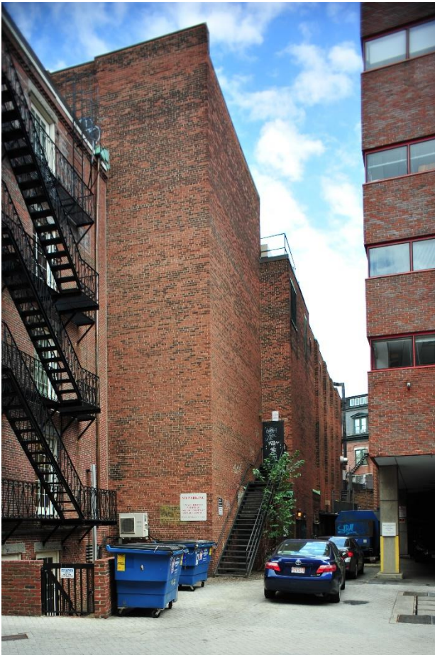
10 Church Street, west and south facades
