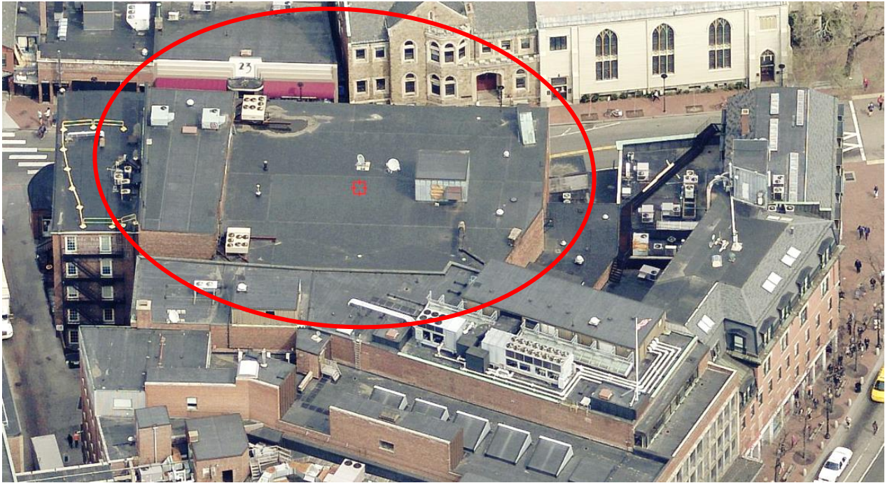
10 Church Street, southerly view, 2014
