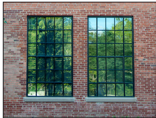
ALUMINUM STEEL REPLICA BLACK TRIM AND MUNTINS DIVIDED LITE WINDOWS
