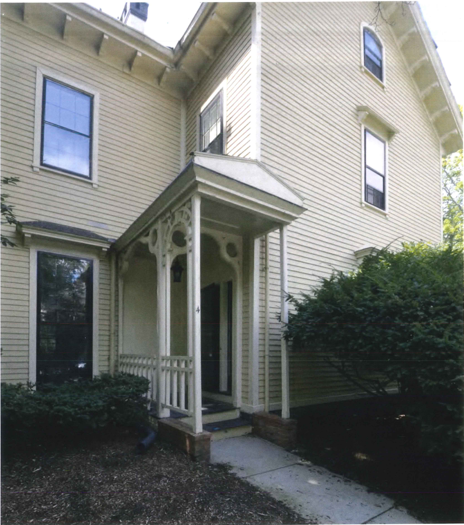
4 Berkeley Street, Lesley University Modifications to porch facing Berkeley Street 12 Feb 19
