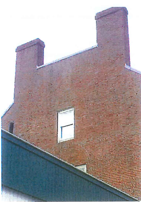
East elevation showing window at attic level
