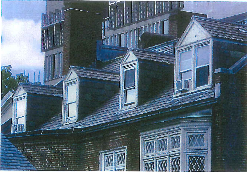
Mix of existing roof slate colors
