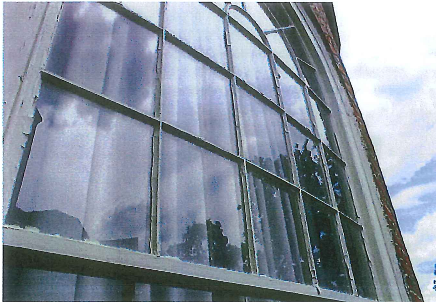
Typical sash conditions of original wood windows
