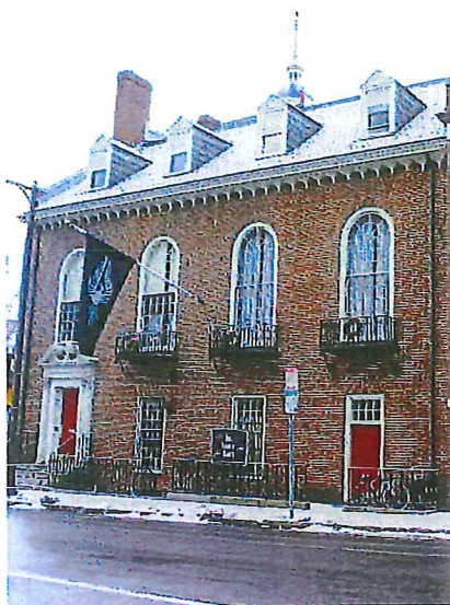
Current conditions, no skylight
