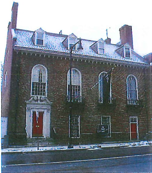
Current conditions, no skylight
