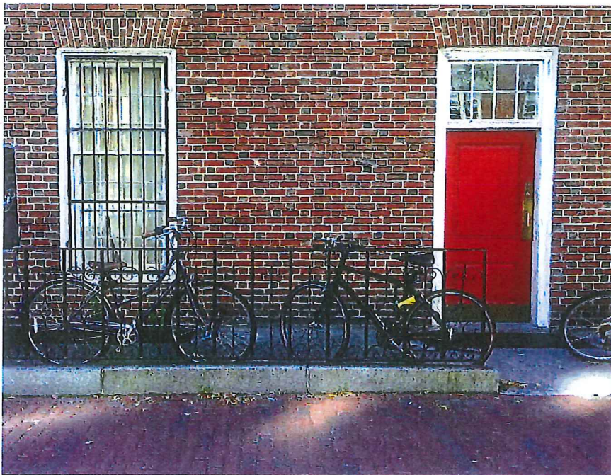
Existing conditions at secondary entrance – proposed for accessibility reconfiguration
