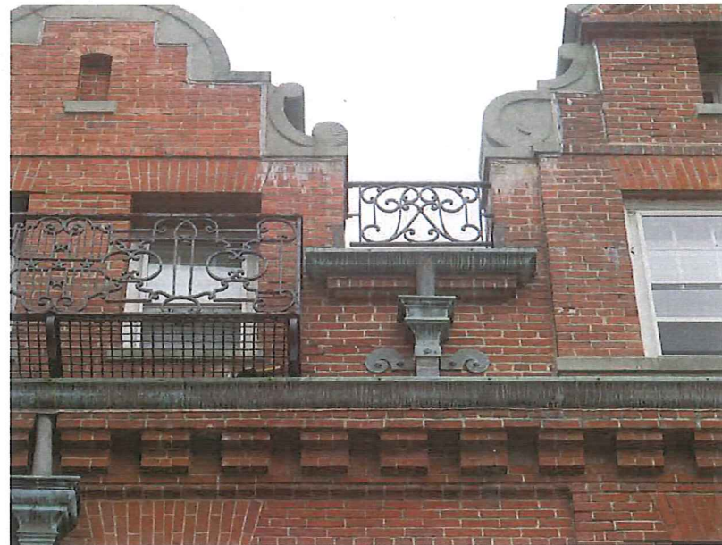
BALCONY AND BALUSTRADE TYPICAL OF EAST & WEST WINGS
