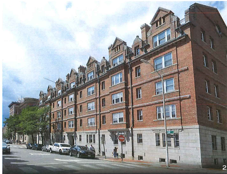
AT PLYMPTON/BOW STREETS - LOOKING NORTHWEST
