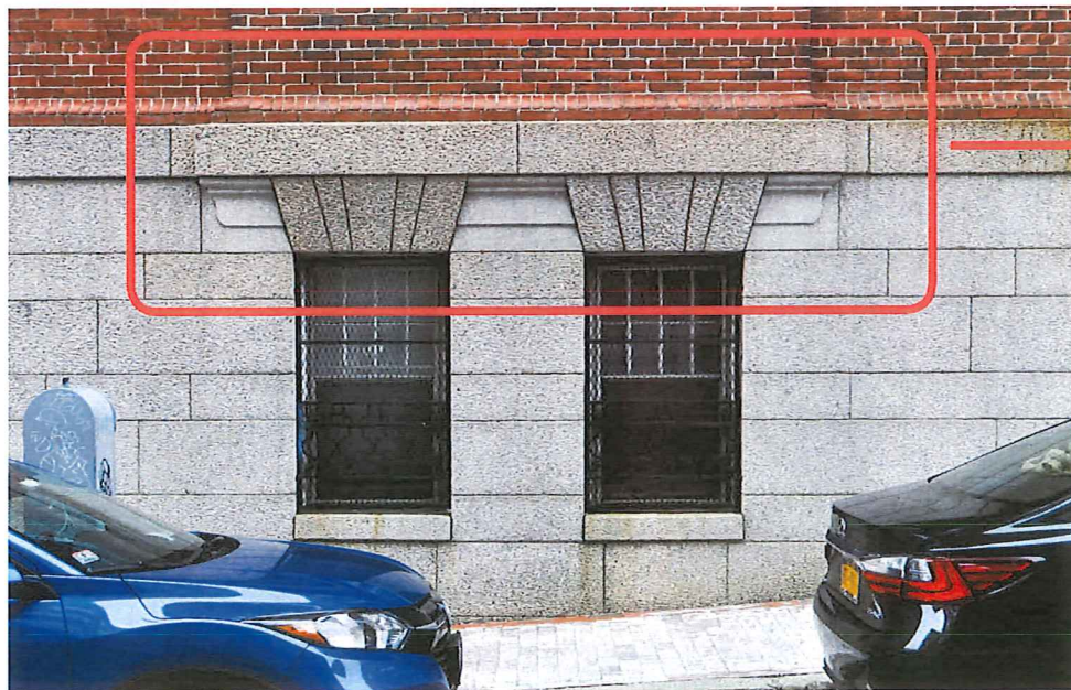
2. PHOTO OF WINDOW HEAD DETAIL - NEXT PROJECTING BAY TO SOUTH
