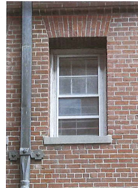
STREET-SIDE DOUBLE-HUNG SASH
