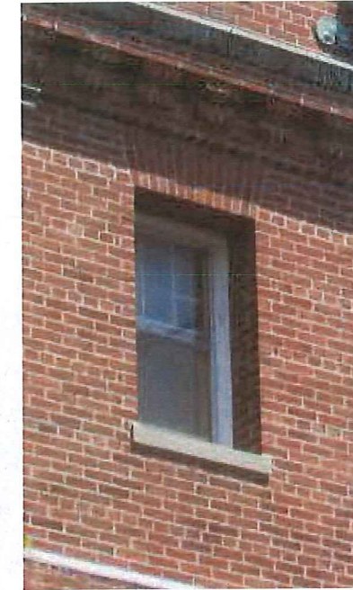
EXISTING WINDOW TYPES - INDIVIDUAL DOUBLE-HUNG SASH WINDOWS (SILL HEIGHTS AND RECESSES VARY)
