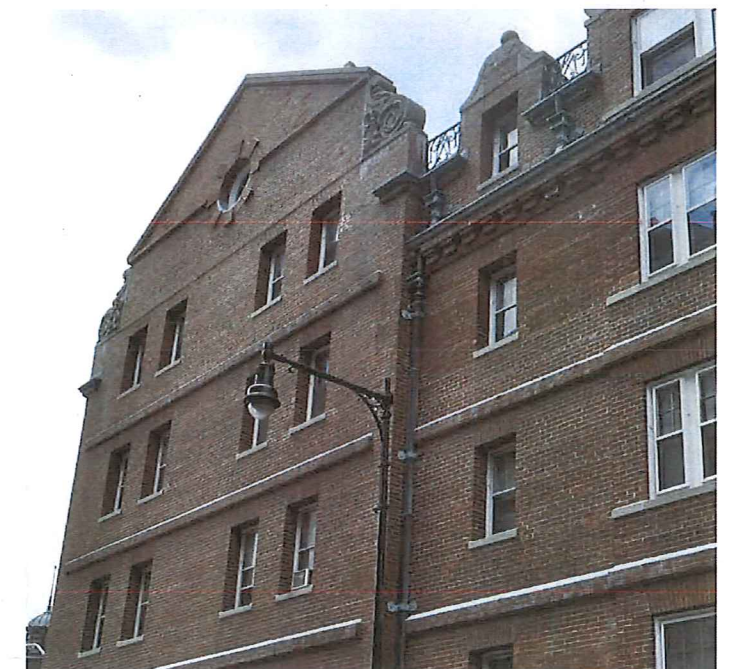
EAST FACADE GABLE-END
