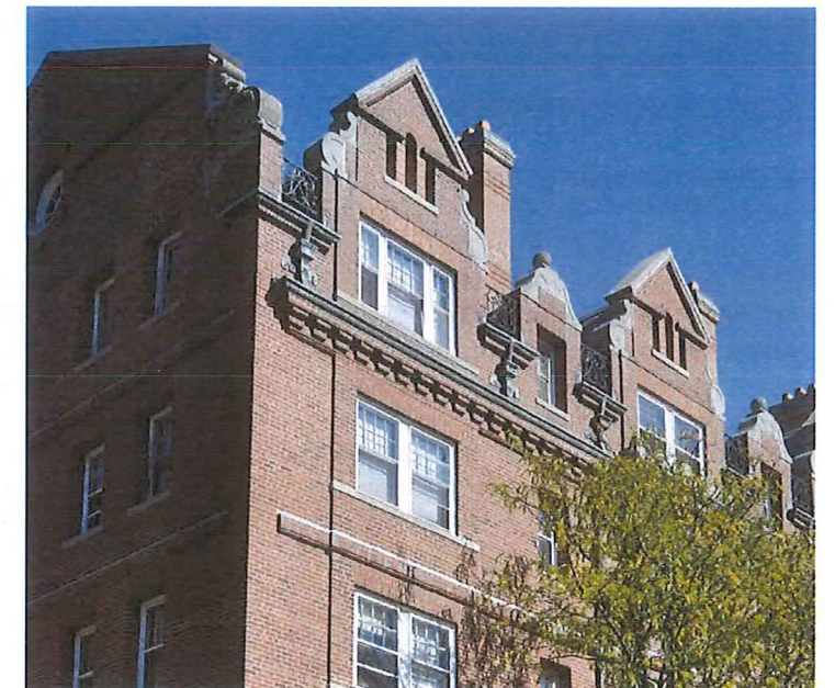
SOUTHWEST CORNER DORMER AND GABLE END
