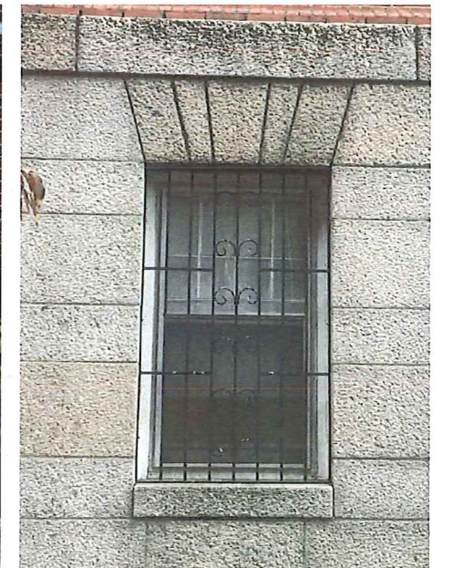
GROUND FLOOR SASH AT WEST WING
