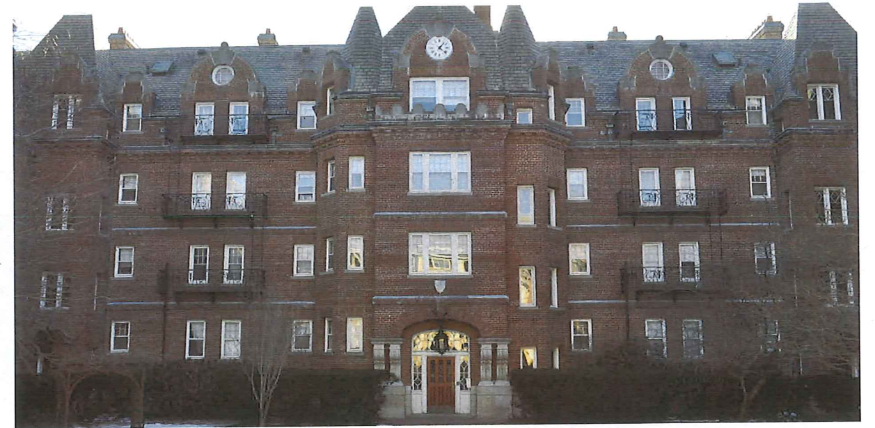
SOUTH COURTYARD BALCONIES WITH UNORIGINAL LADDERS AND WIDTH EXTENSIONS
