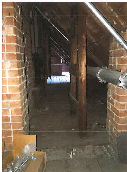
ATTIC SPACE IS INSUFFICIENTLY LARGE TO FIT MECHANICAL EQUIPMENT
