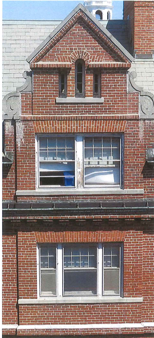
MULTI DIVISION WINDOWS AT WEST WING
