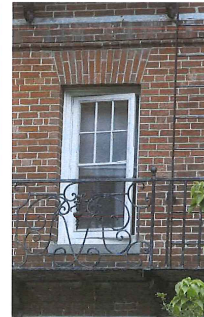
CASEMENT AT BALCONY
