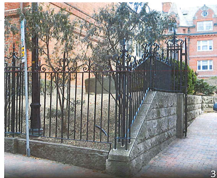
RETAINING WALL AT LINDEN ST ENTRY TO COURTYARD
