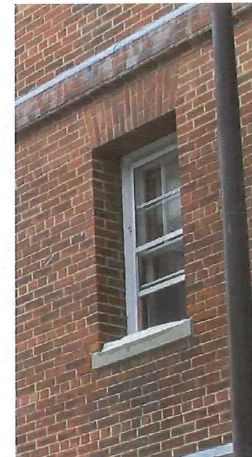
EXISTING WINDOW TYPES - INDIVIDUAL DOUBLE-HUNG SASH WINDOWS (SILL HEIGHTS AND RECESSES VARY)
