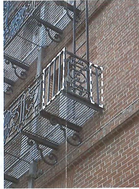
WEST WING BALCONIES - NOTE NON-ORIGINAL ALTERATIONS TO BALCONY BE REMOVED, SHOWN WITH WHITE DASHED LINES AT RIGHT
