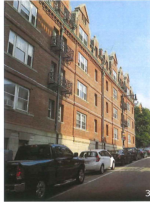
VIEW NORTH ON PLYMPTON ST
