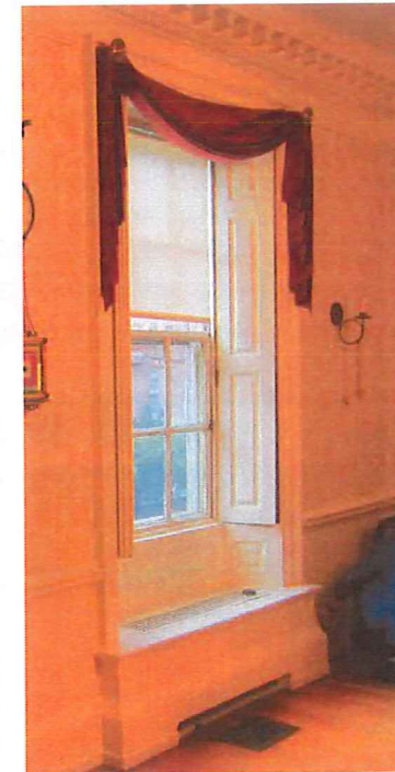
EXISTING WINDOW INTERIOR WITH ORIGINAL POCKETED SHUTTERS
