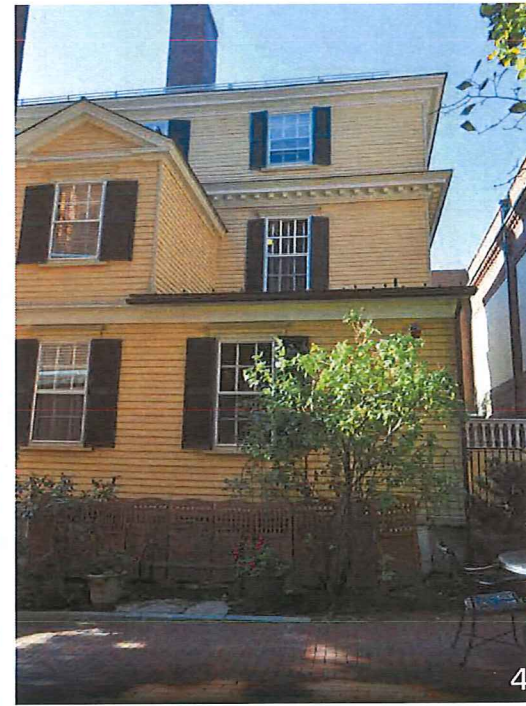
VIEW OF EAST FACADE (LOOKING WEST)
