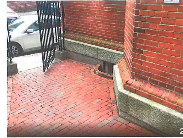
PLYMPTON GATE LOOKING SE
