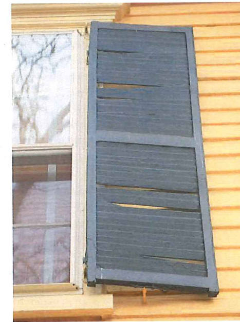
SHUTTER DETERIORATION
