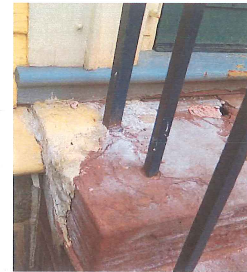
STOOP CONDITIONS - DETERIORATING SANDSTONE STEPS WITH VOIDS
