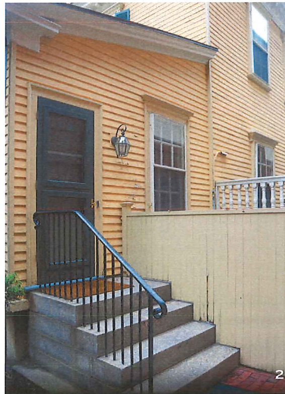
EXISTING CONDITIONS NORTH ENTRY
