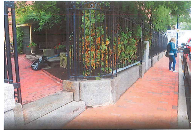
PLYMPTON STREET FENCE AND RETAINING WALL
