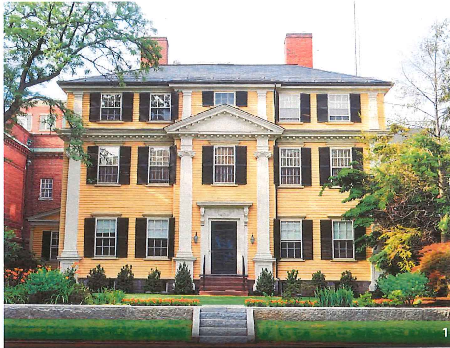
SOUTH (PRIMARY) FACADE VIEWED FROM RANDOLPH COURTYARD
