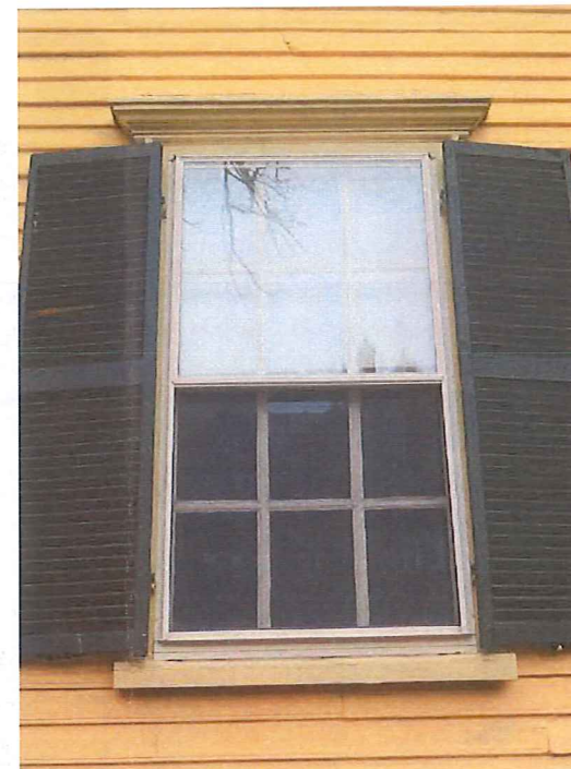
TYPICAL EXISTING SASH WINDOW
