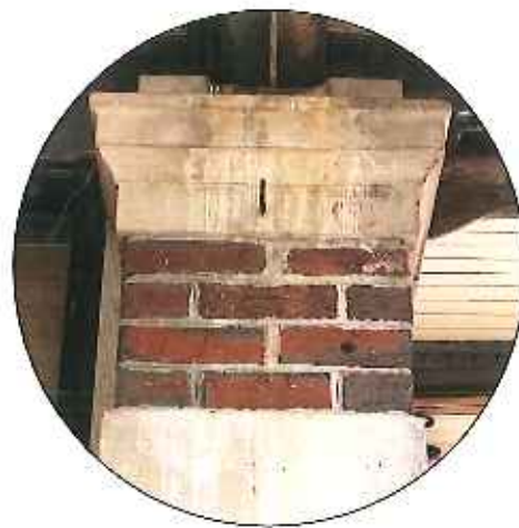
anchor / remove and patch
