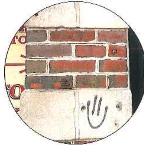
anchors / remove and patch hole / patch
