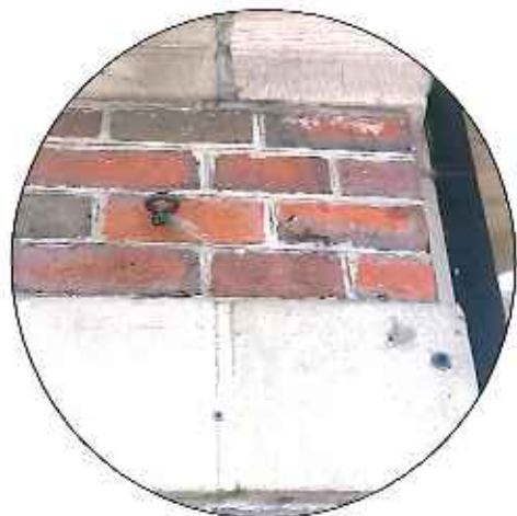
anchors / remove and patch hole / patch
