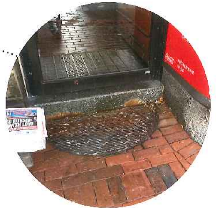
present day entry - west
