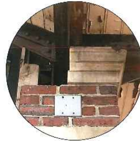
limestone return missing / replicate
