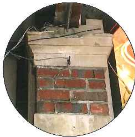
anchor / remove and patch limestone spall / dutchman
