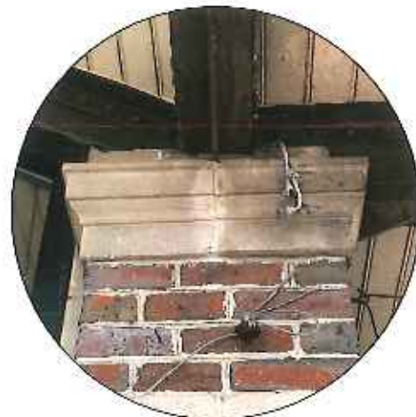
4 anchor / remove and patch
