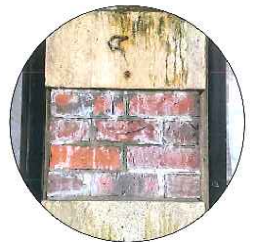
anchors / remove and patch area of repeated water saturation and biological growth
