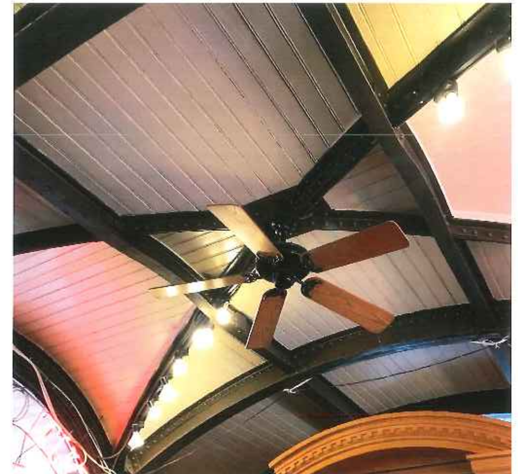
soffit today - dark steel, light soffit
