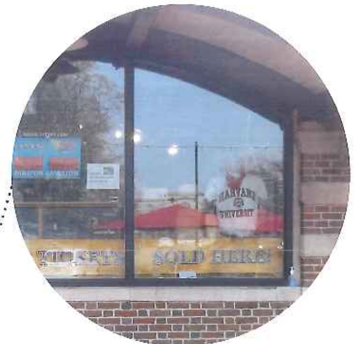
restore glass with thin dimensions of the original mullions.
