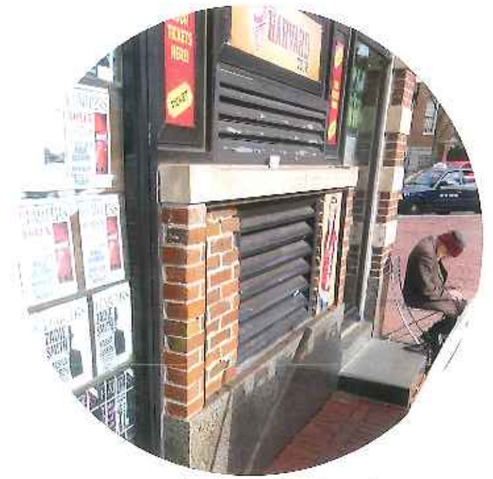
vents along south elevation
