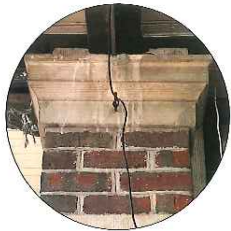
anchor / remove and patch
