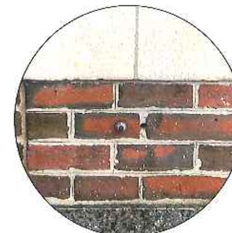
7 anchor / remove and patch
