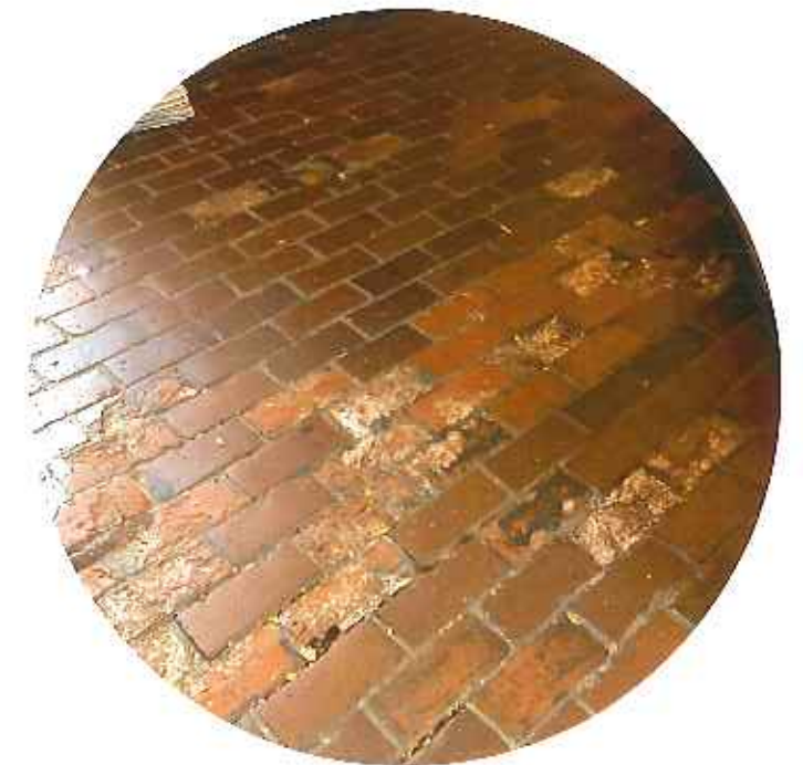
address MAAB compliant brick floor
