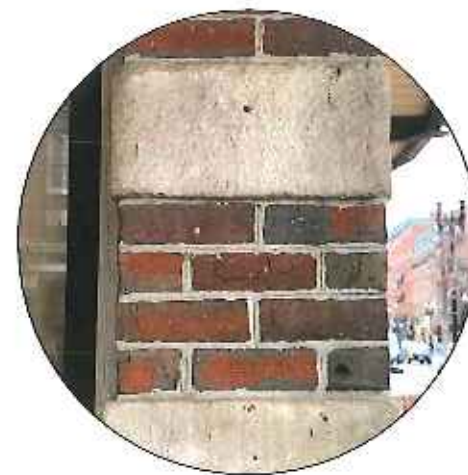
anchors / remove and patch hole / patch
