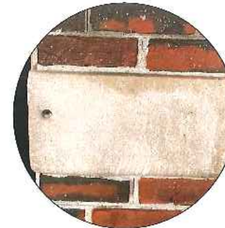
4 anchor / remove and patch
