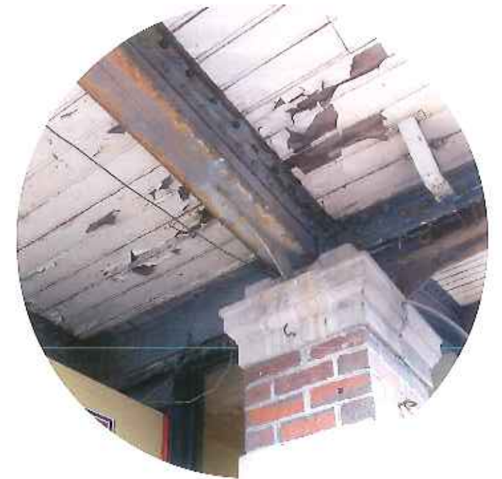
restoration / replacement of exposed beadboard
