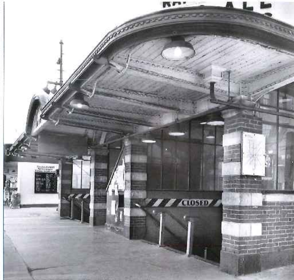
renovated soffit - light color
