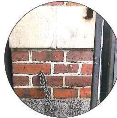
anchors / remove and patch
