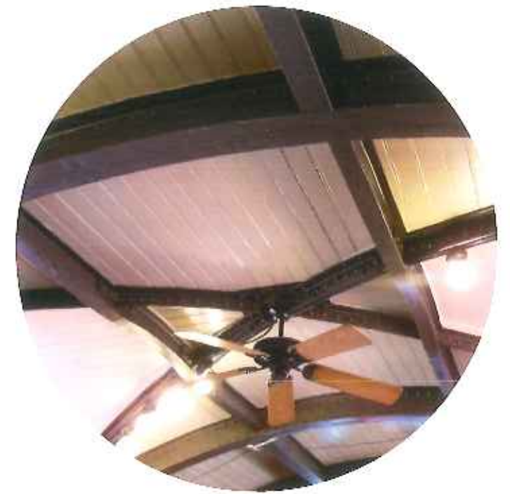
preserve exposed wood beadboard & riveted iron structure
