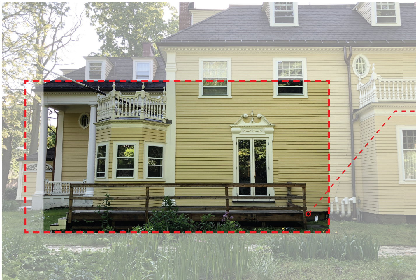
1 EXISTING CONDITION - SIDE PORCH L6.0 SCALE: NTS
