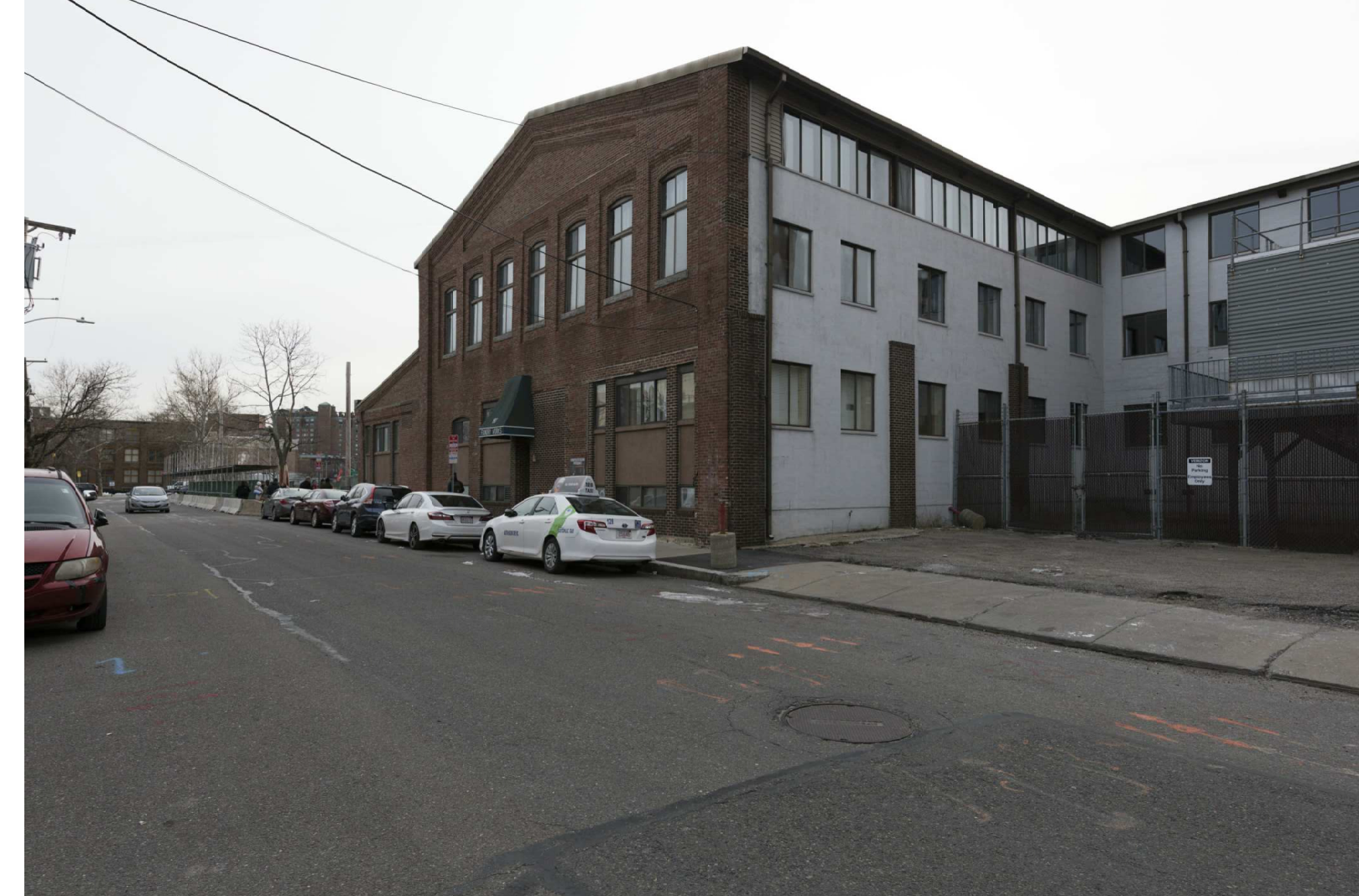
BENT STREET TOWARDS THIRD STREET
