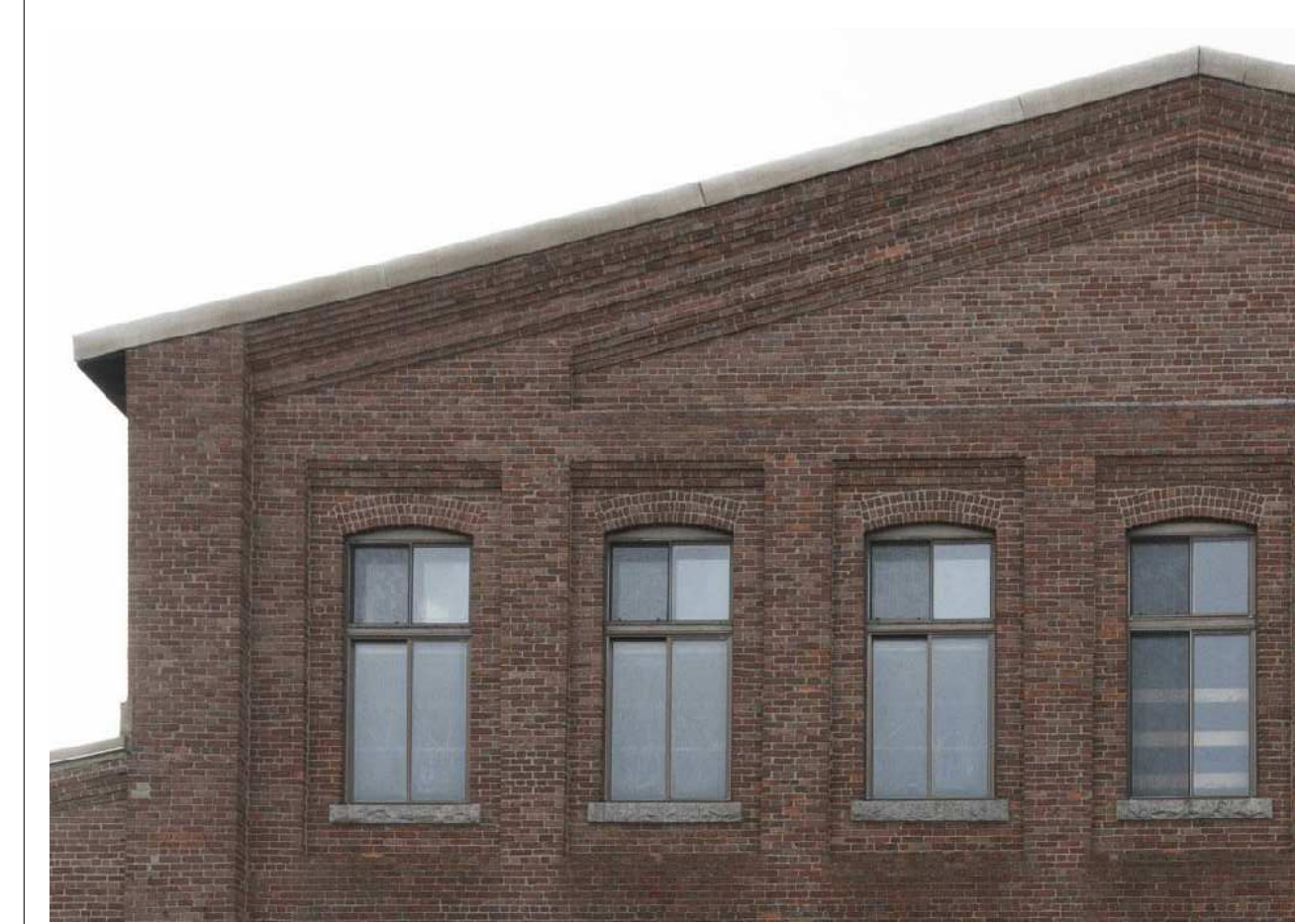
EXISTING CONDITION - TYPE 3
