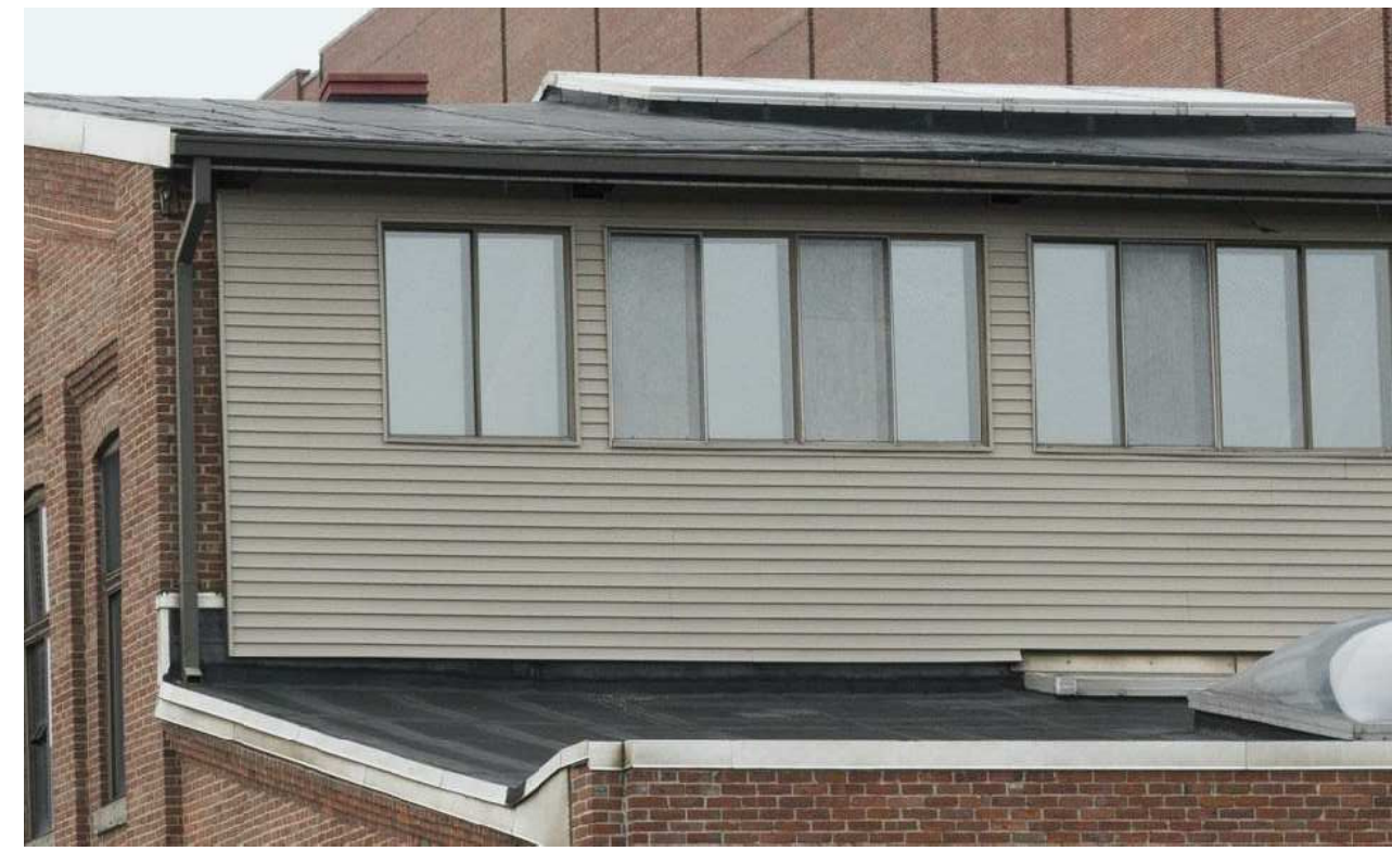
EXISTING CONDITION - TYPE 4
