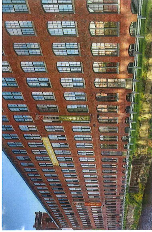
Replacement window system: two views of the proposed "Universal" 400 aluminum window system, with heavy mullions and applied muntins, in Kynar paint finish as used at two other Massachusetts renovation projects. Operable sash are not proposed.
