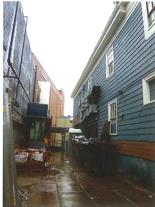
VIEW OF EXISTING SERVICE ALLEY AND MECHANICAL EQUIPMENT TO BE REMOVED
