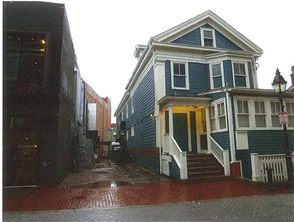
VIEW IS SOUTH FROM WINTHROP STREET, SERVICE ALLEY IS TO THE LEFT
