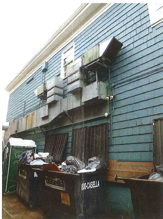
VIEW OF EXISTING MECHANICAL EQUIPMENT TO BE REMOVED
