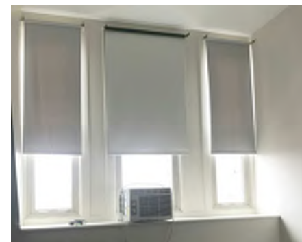
EXISTING DORMER #1 - INTERIOR PHOTO
