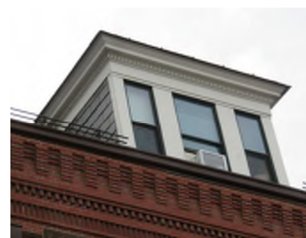
EXISTING DORMER #1 - EXTERIOR PHOTO
