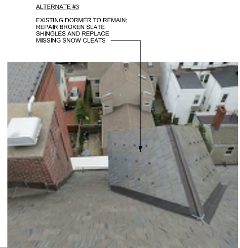
EXISTING DORMER #1 - ROOF PHOTO
