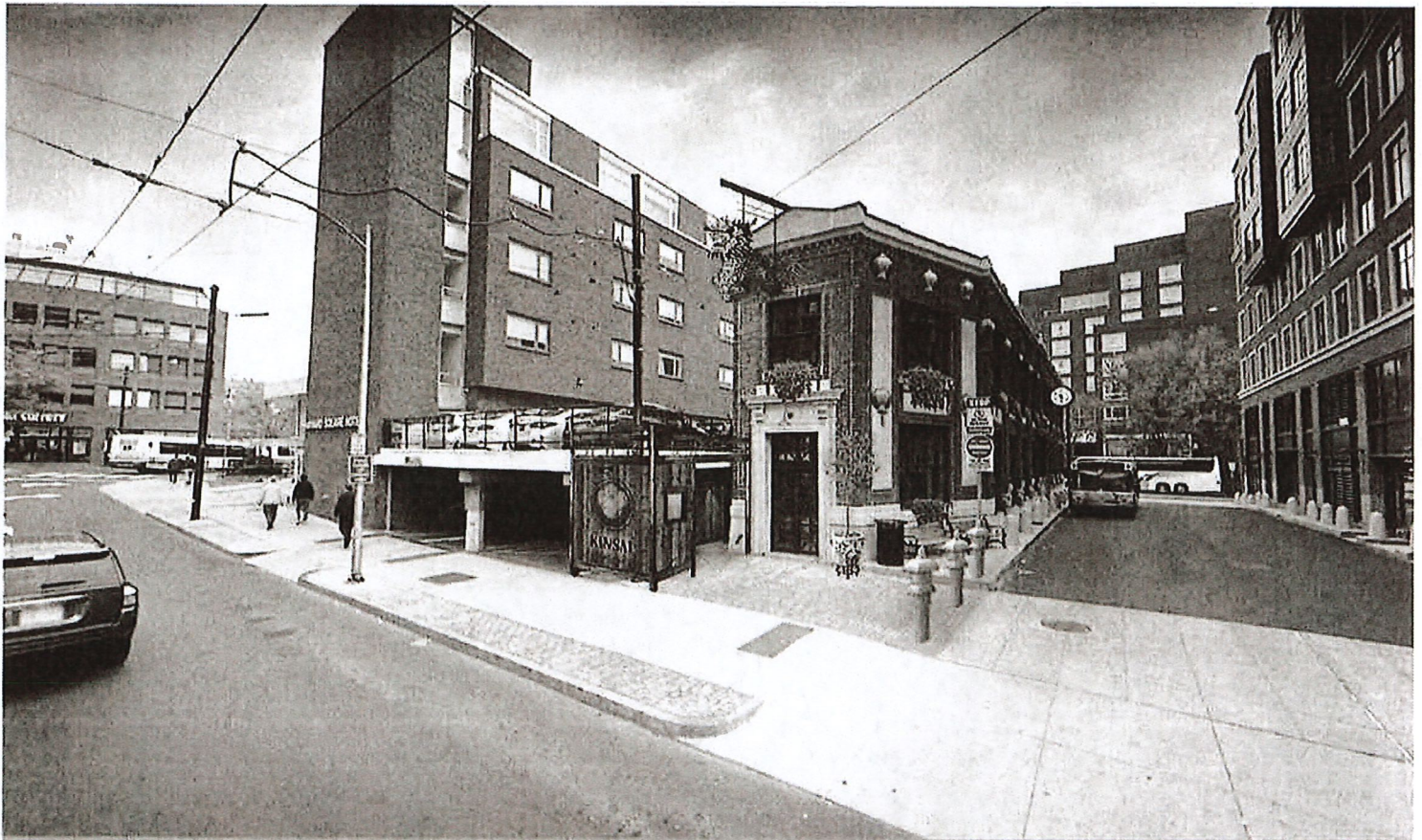
EXTERIOR DESIGN / MOUNT AUBURN STREET VIEW
