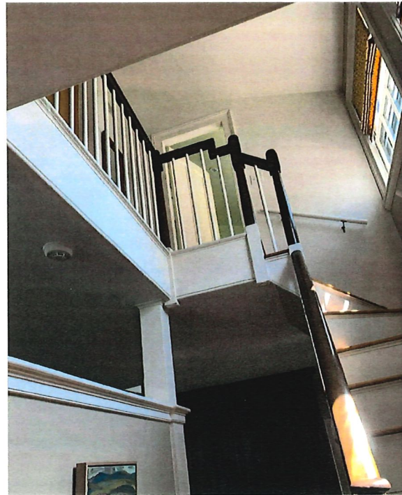
1 DANGEROUS WINDER CONDITION AT EXISTING BACK STAIR TO 2ND FLOOR NTS
