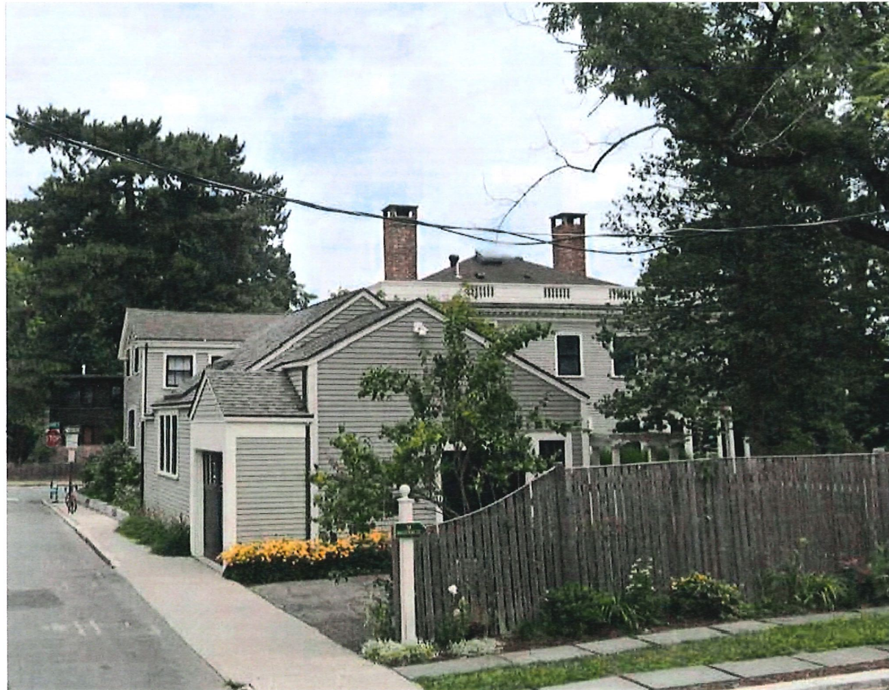
1 VIEW FROM MADISON STREET - EXISTING NTS
