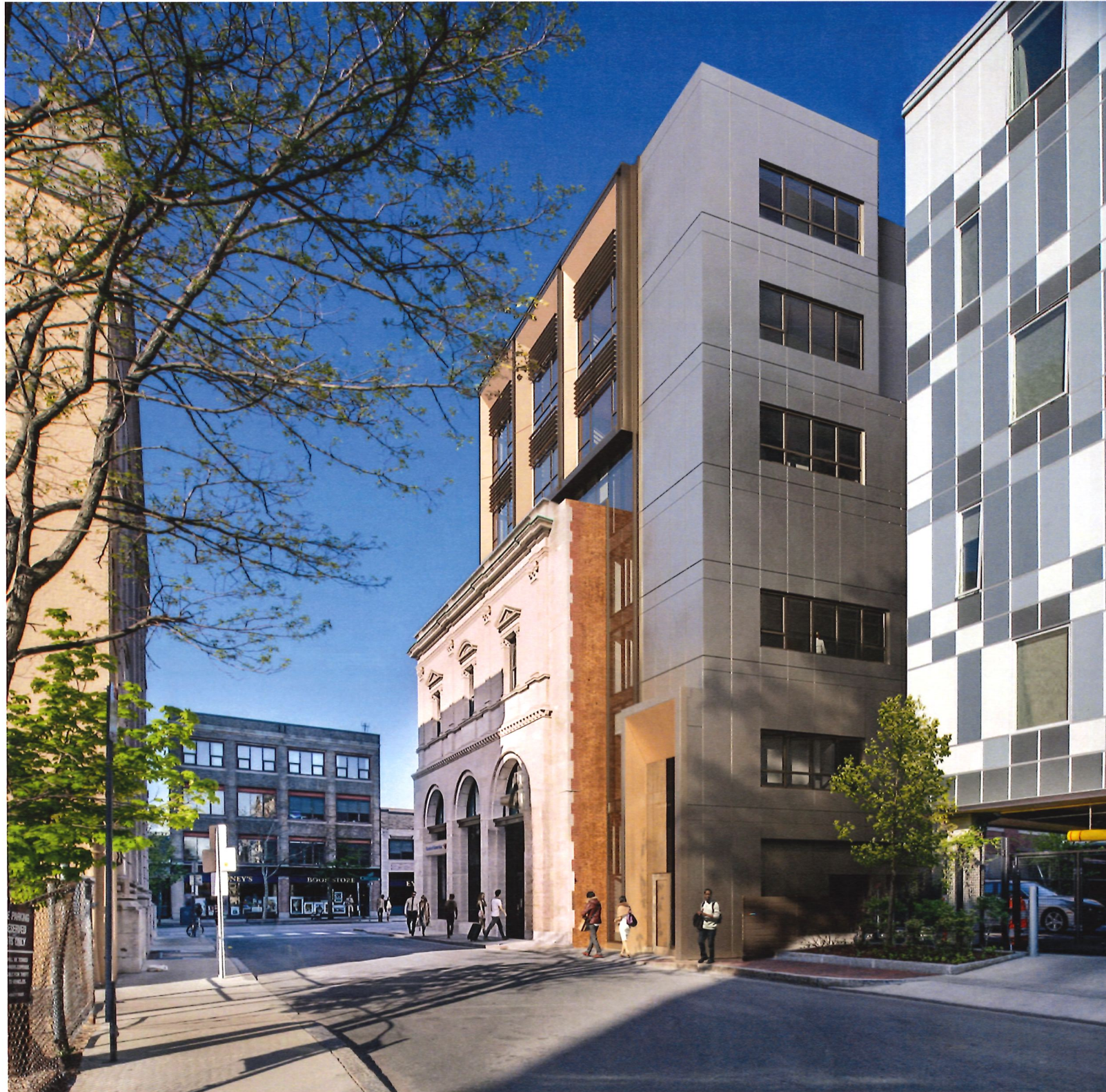
5A View of Hotel Entry From Temple Street - Near
