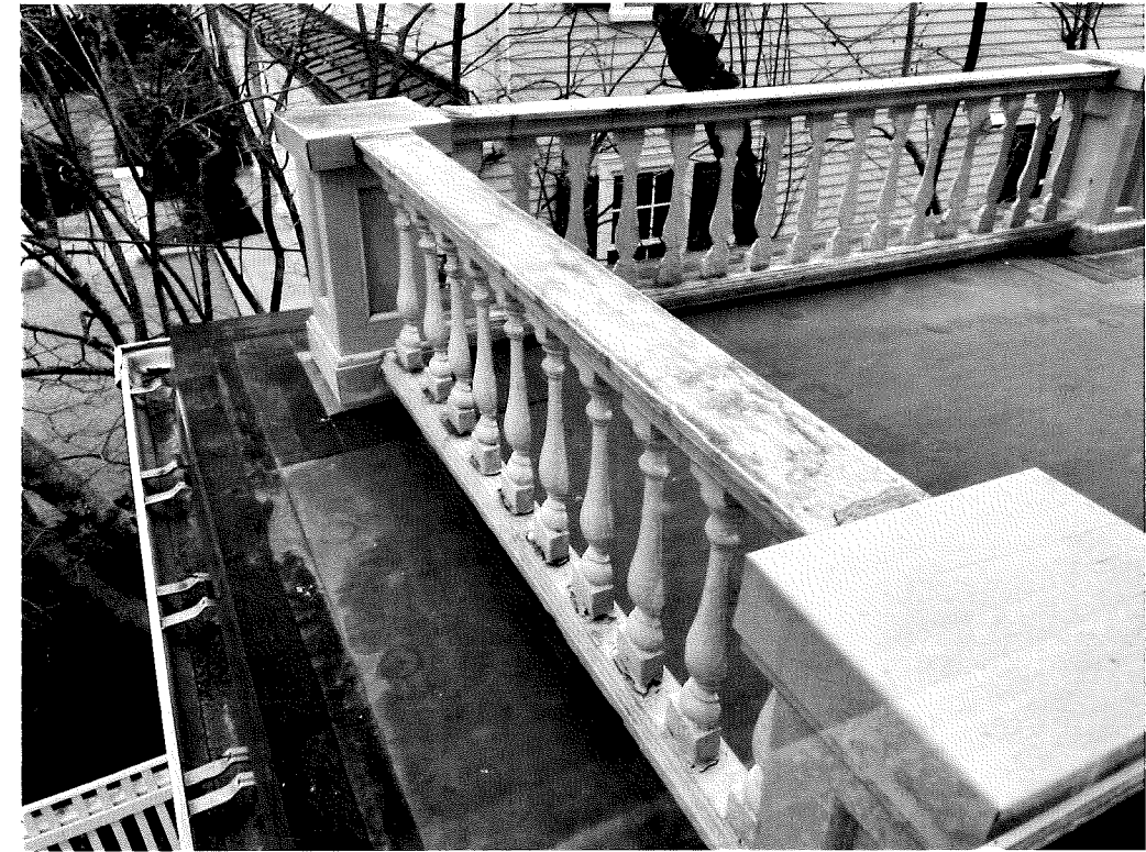
RAILING ON RIGHT OF HOUSE
