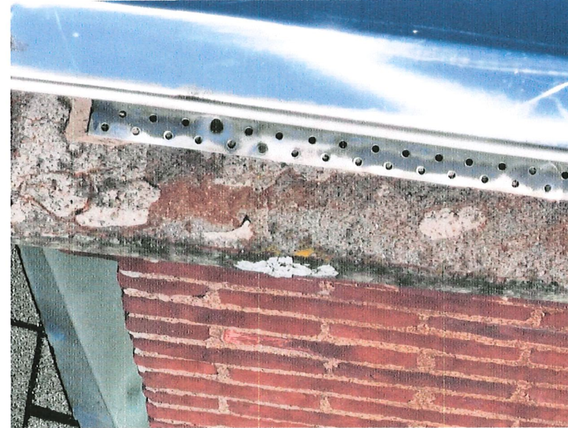
CURRENT SITE CONDITIONS - CHIMNEY DETAIL DATE: 2023
