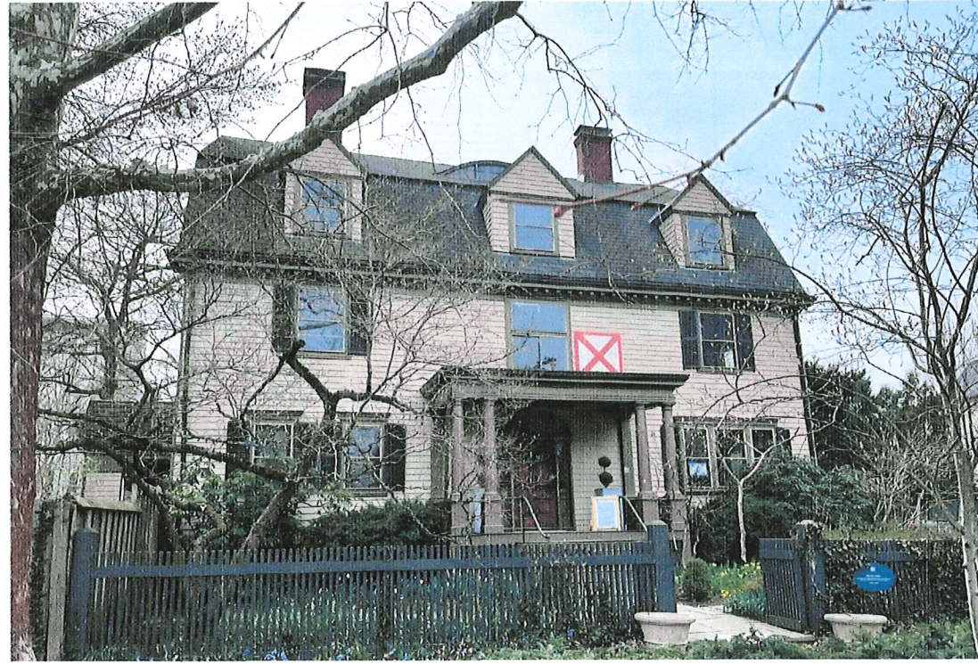
CURRENT SITE CONDITIONS (VIEW FROM IRVING STREET) DATE: 2023
