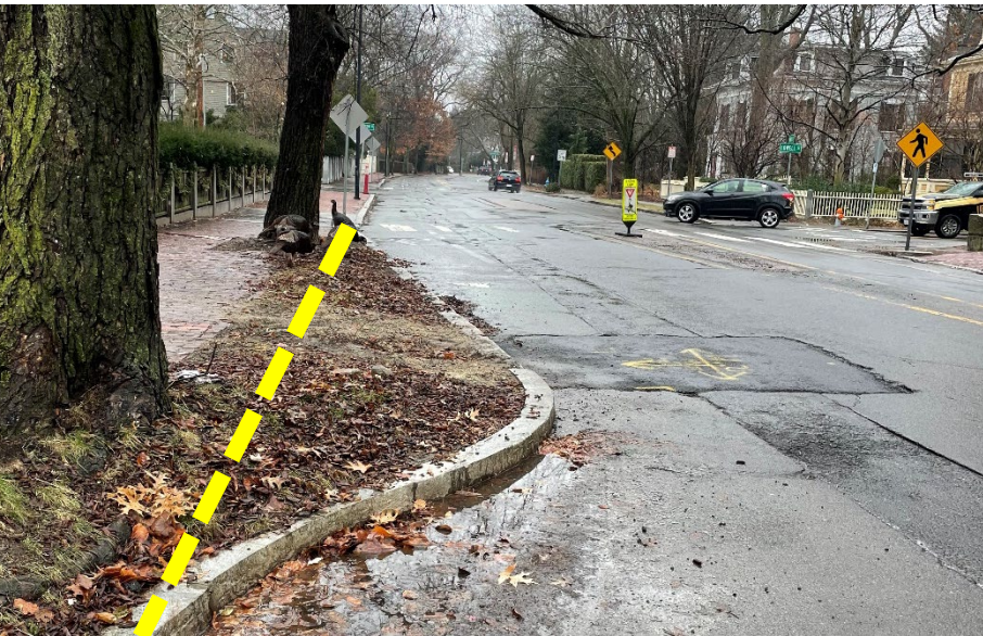
Photo of an existing curb bump out
