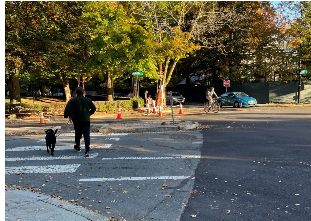
Existing Pedestrian Crossing island at Brattle St and Sparks St to be removed
