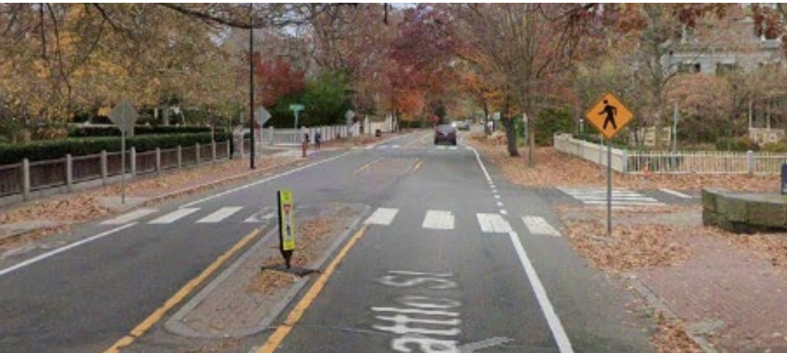
Existing flush crossing island, which does not protect people from traffic
