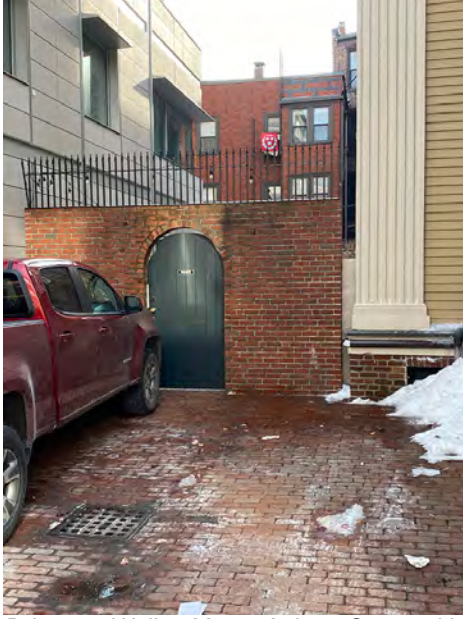
Driveway Wall at Mount Auburn Street with Gate & Guard Similar to JFK Garden Wall
