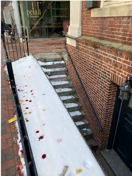
Areaway Stairs Parallel to North Facade at Mt. Auburn
