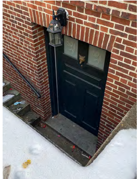
Basement Door in North Facade Areaway
