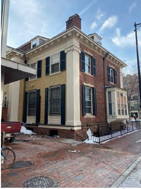
View of Fox Club from Mount Auburn Street; North & South Facades are Brick; East & West Facades are Painted Wood Clapboards
