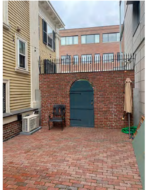
Driveway Wall with Wooden Gate and Metal Guardrail to Match JFK Garden Wall
