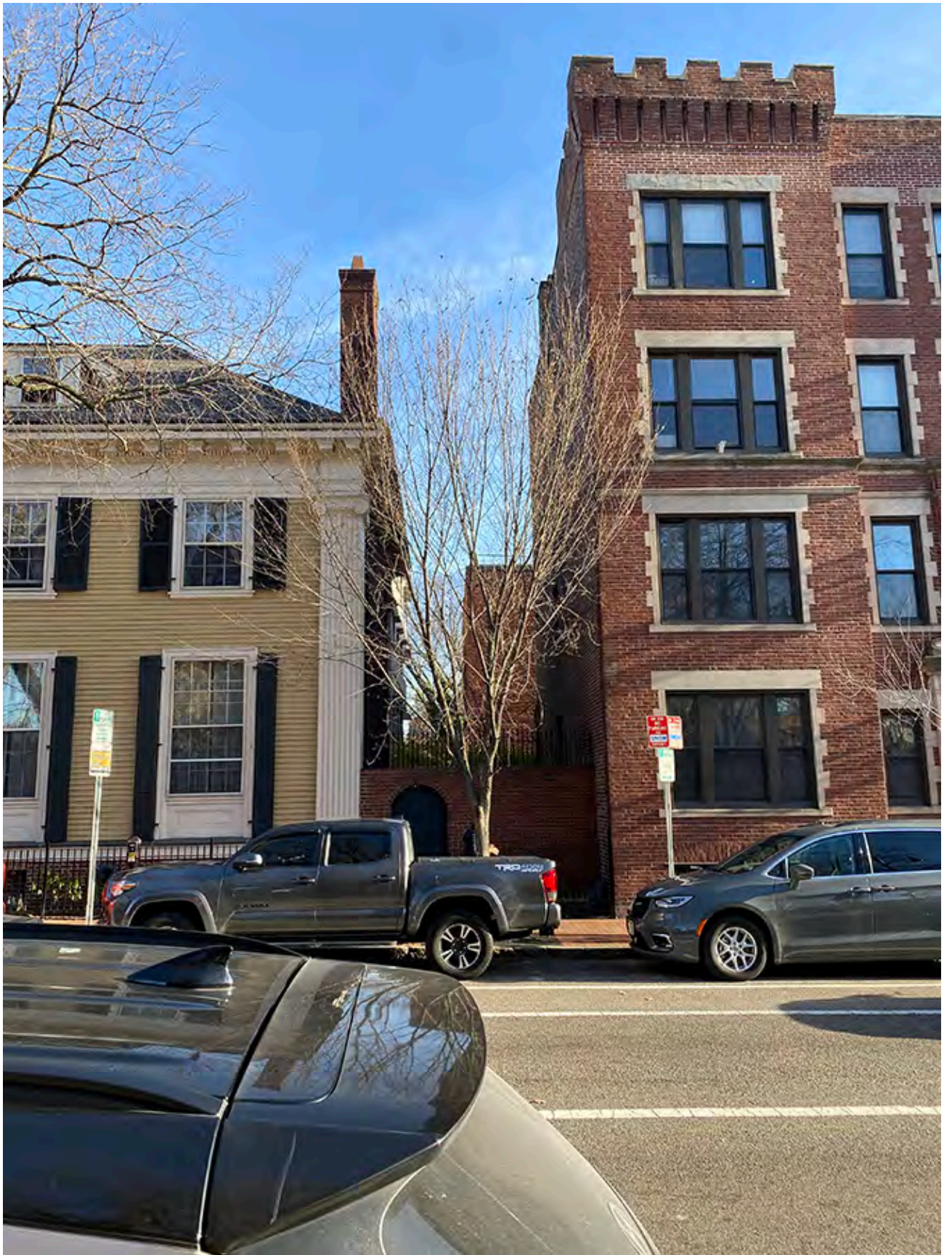
Interstitial Sideyard Space Between the Fox Club and Adjacent 48 JFK Apartment Building
