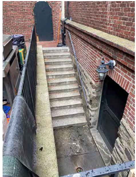
Areaway Stairs to Basement from Sideyard; Gate at Garden Wall Beyond
