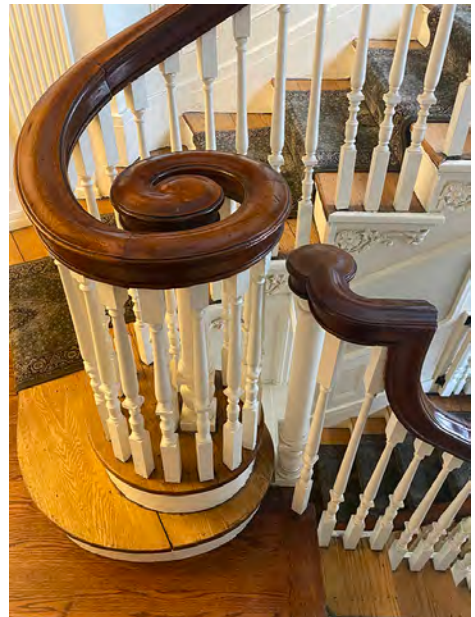
Details at Original First Floor Stair Balustrade
