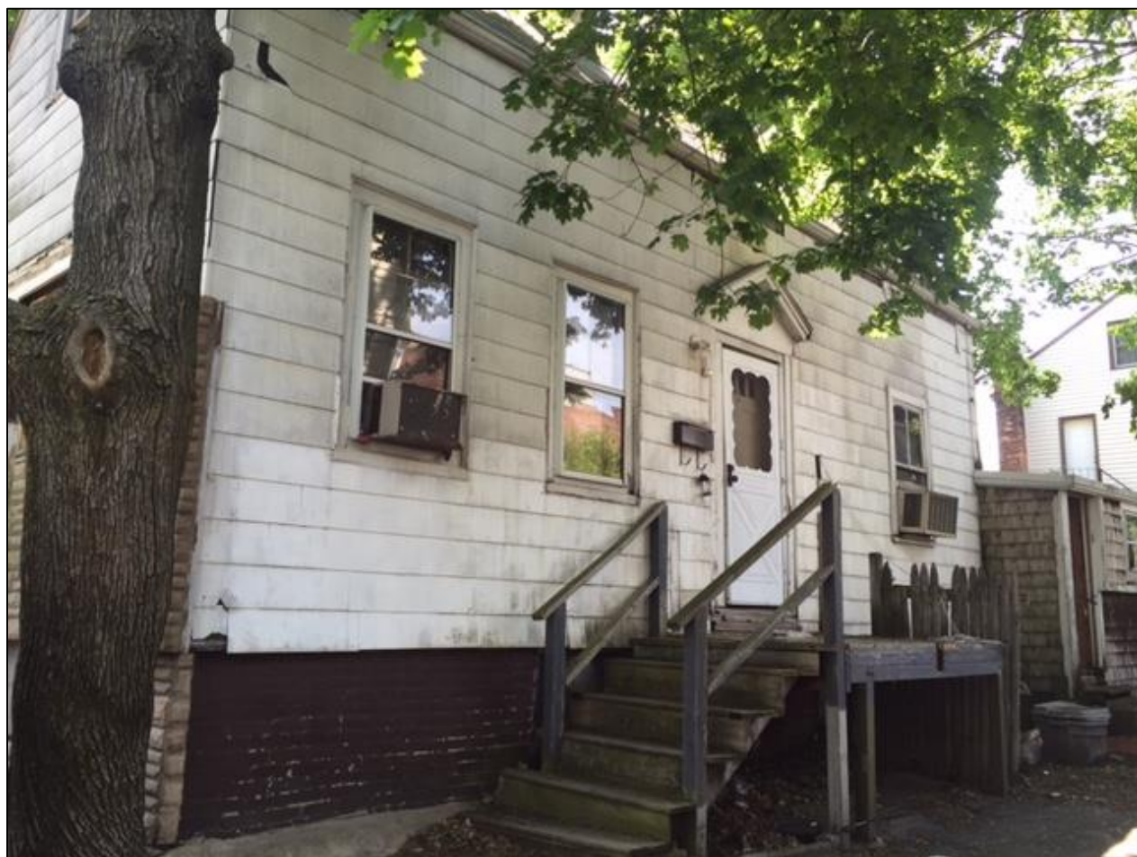
86 School Street, front (west) elevation with shingled 1-story shed addition visible at rear, 2016
