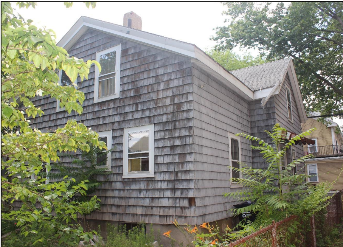
Rear of 146-148 Pearl St., 2016
