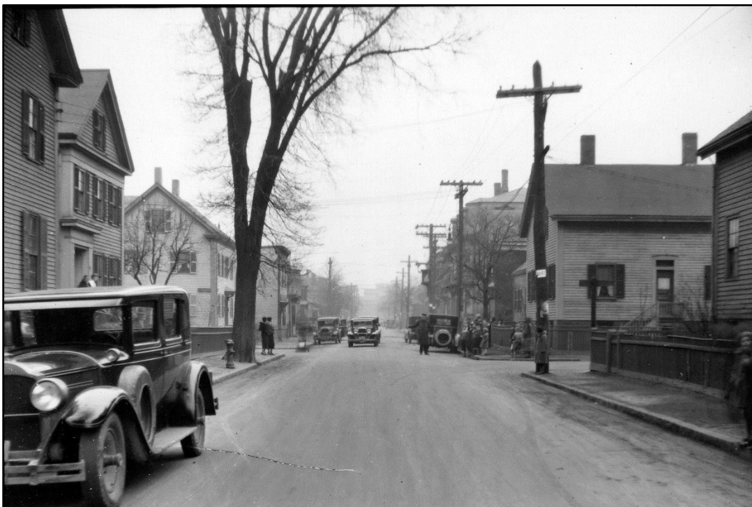
Pearl at Decatur, 1932. Engineering Dept. Collection, CHC Two double workers' cottages at 132 and 138 Pearl Street are visible at the right in this photo.
