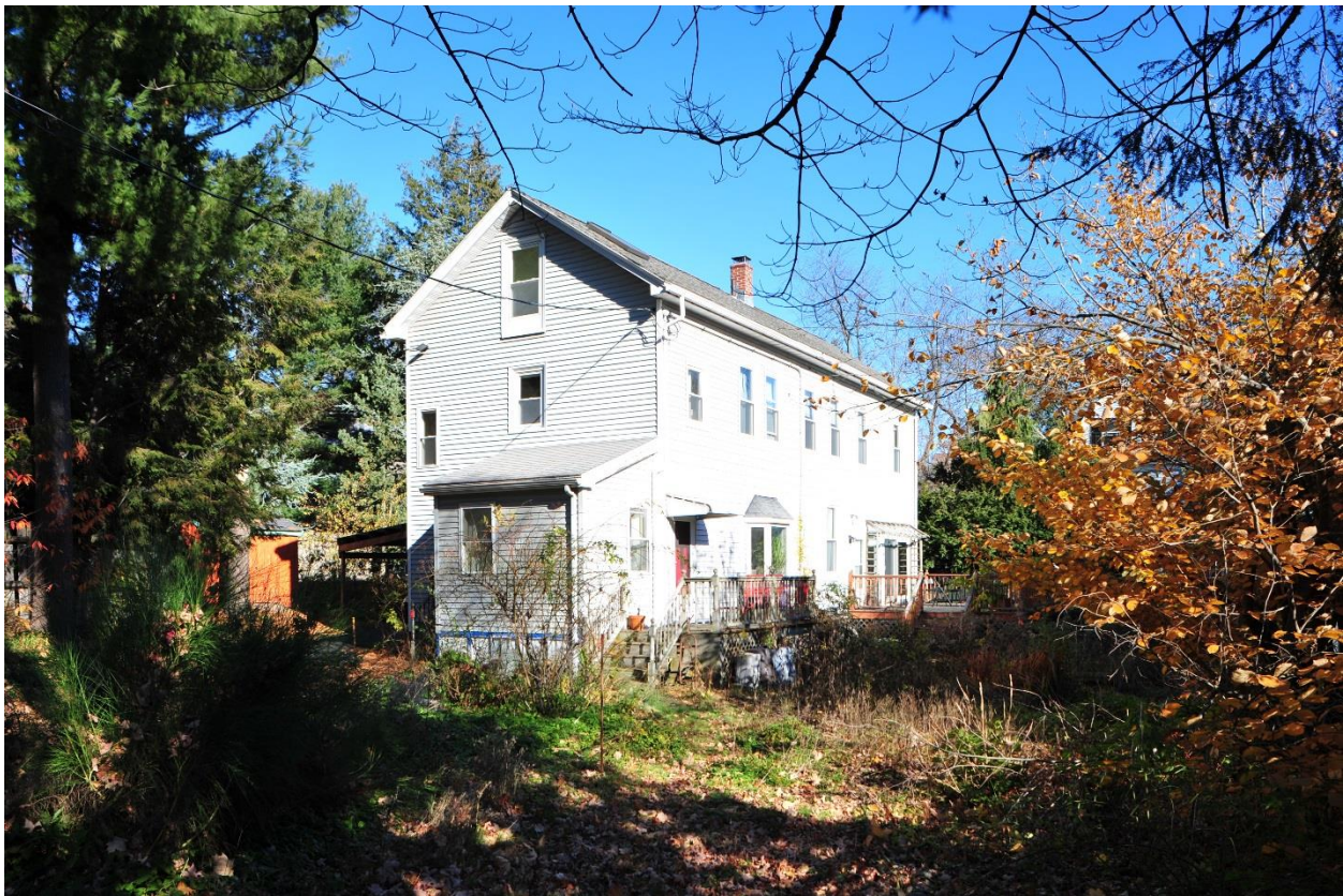
16 Kennedy Road, south and west elevations
