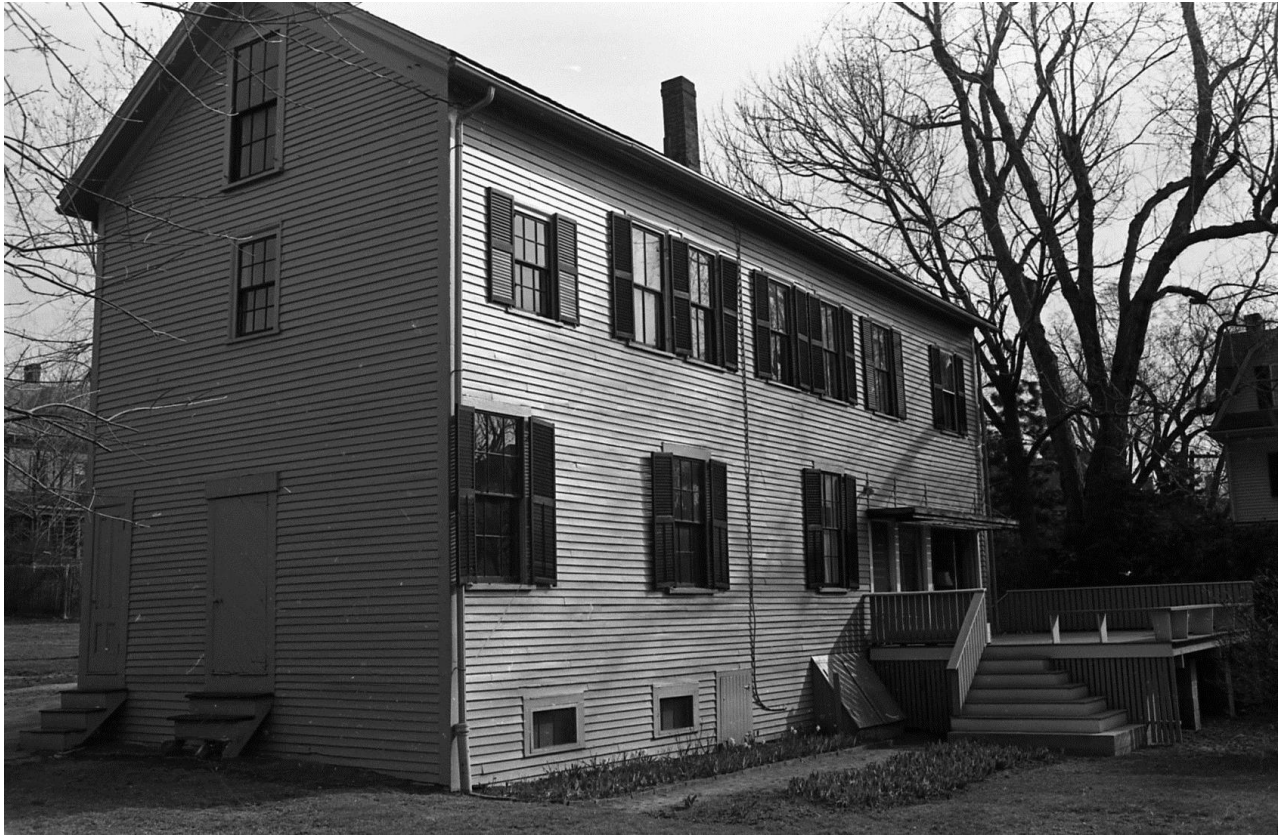
16 Kennedy Road, south and west elevations
