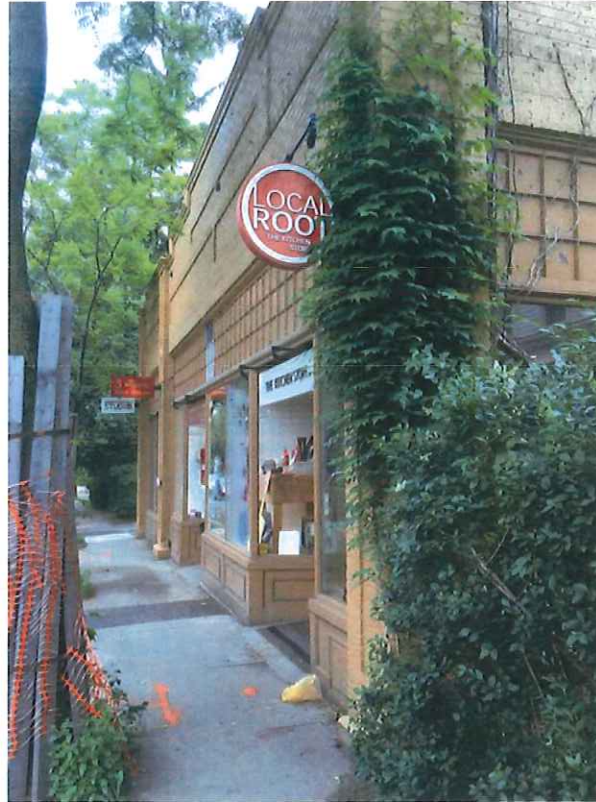
221-225 CONCORD AVE EXISTING RETAIL
