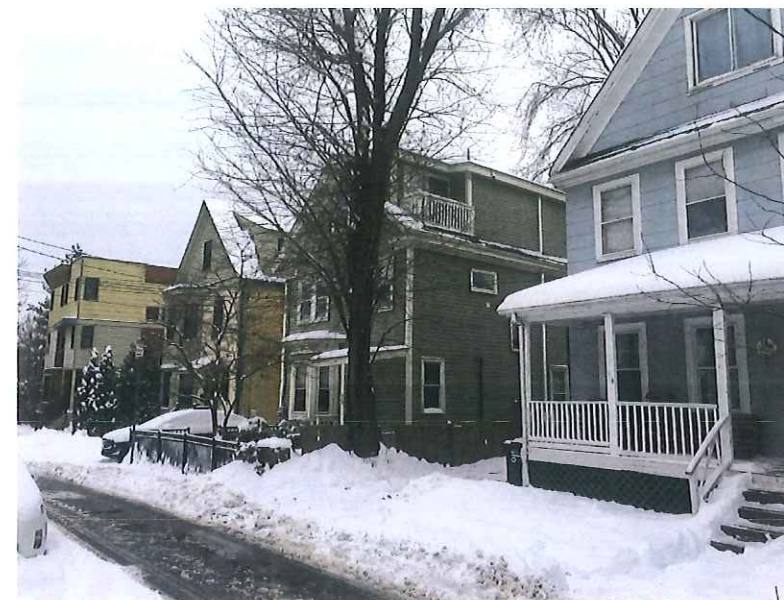
Existing North West View
