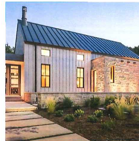
MATCHING STANDING SEAM VERTICAL PANELING AT EAVES
