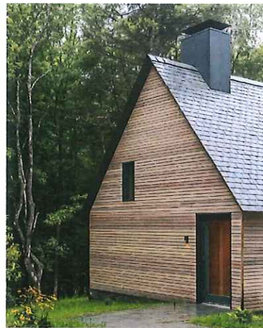
CEDAR SIDING WITH BLACK FENESTRATION
