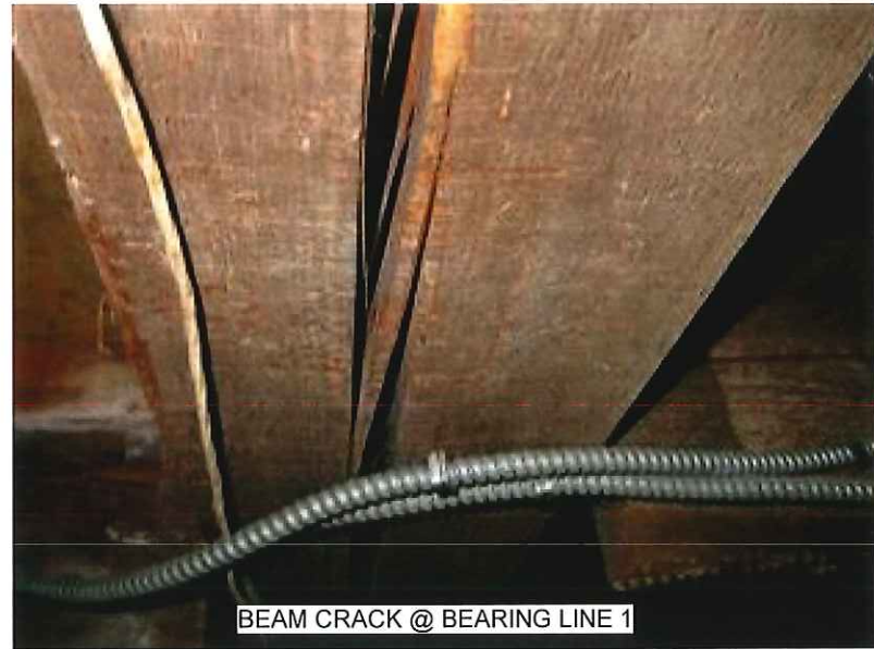
BEAM CRACK @ BEARING LINE 2/C
