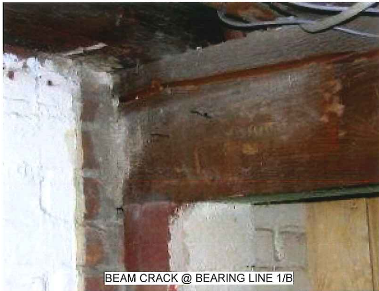
BEAM CRACK @ BEARING LINE B
