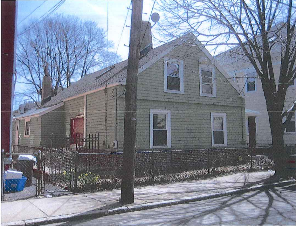
4. 64 Pearl St., front and left side elevations, April 2009. Photo by P. Trudeau
