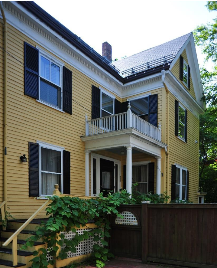
25 Walker Street, front door and porch detail
