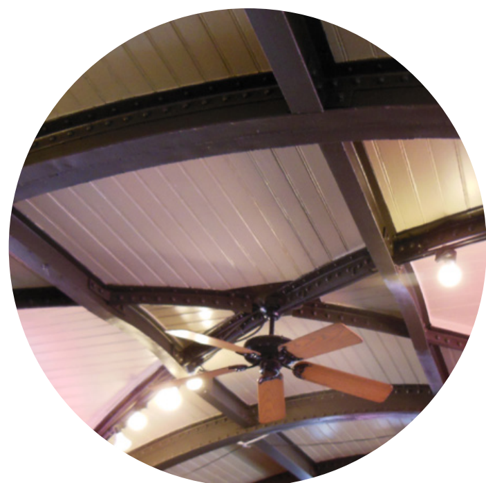
preserve exposed wood beadboard & riveted iron structure
