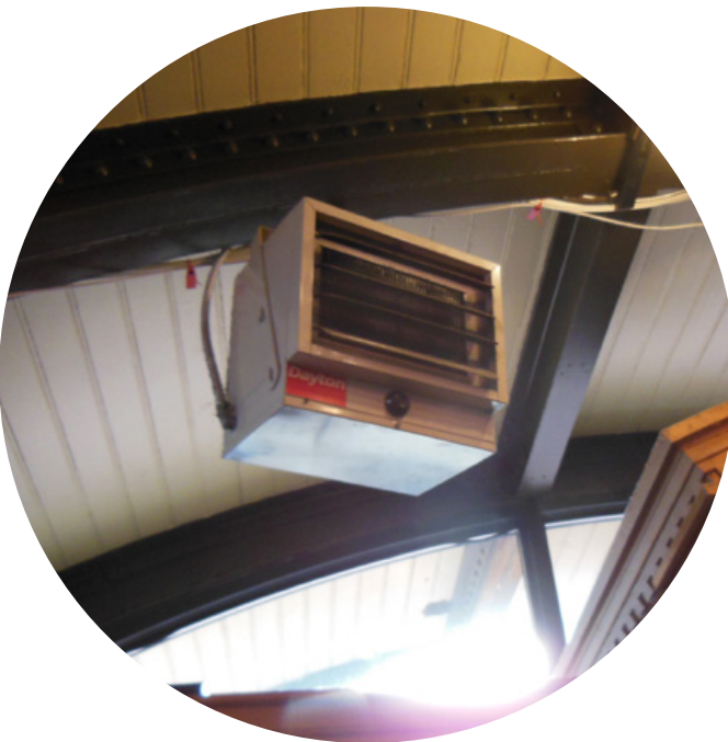
removal of all interior & exterior heating and cooling units for redesign of systems for greater efficiency
