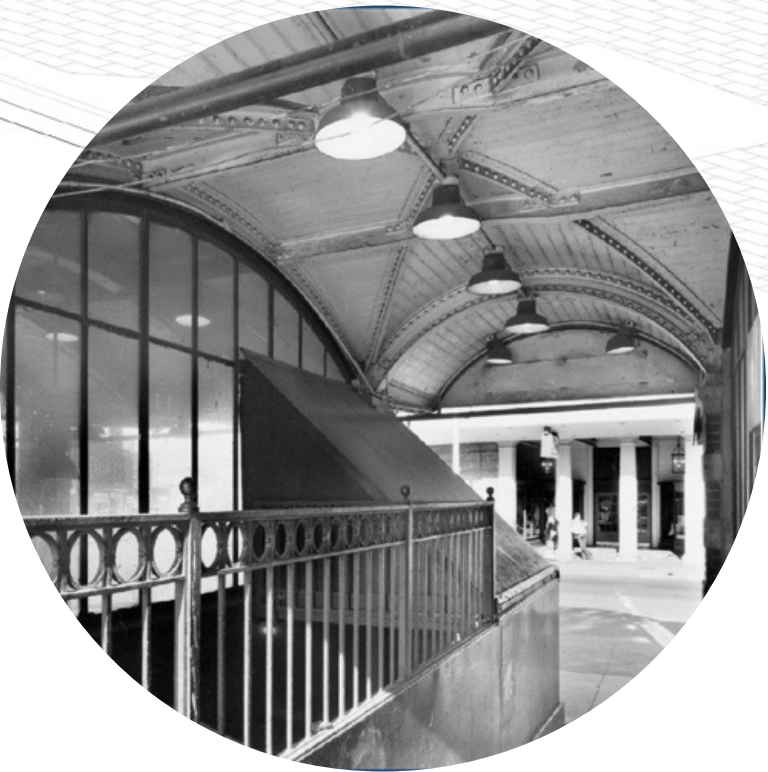
original breezeway - 1977 HARVARD SQUARE KIOSK - CAMBRIDGE, MASSACHUSETTS JULY 12, 2018
