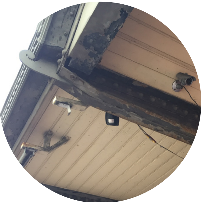
clean structural members for removal of rust and paint, to be repainted in the historic color
