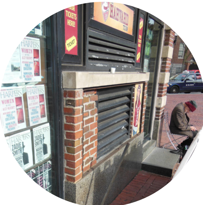
vents along south elevation
