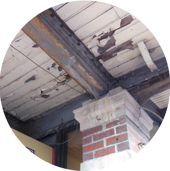
restoration / replacement of exposed beadboard
