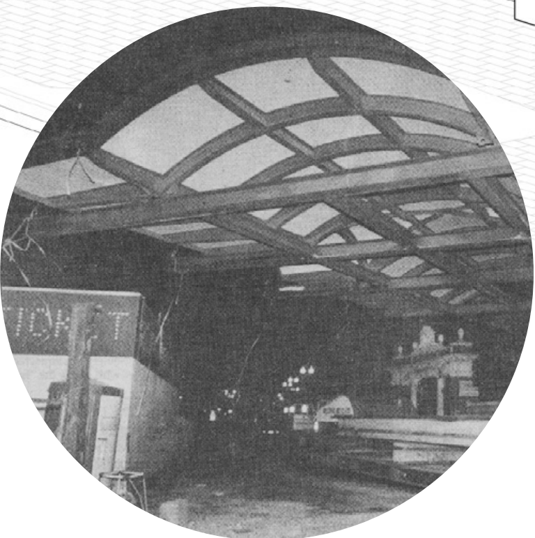
re-installation of original kiosk roof - 1983
