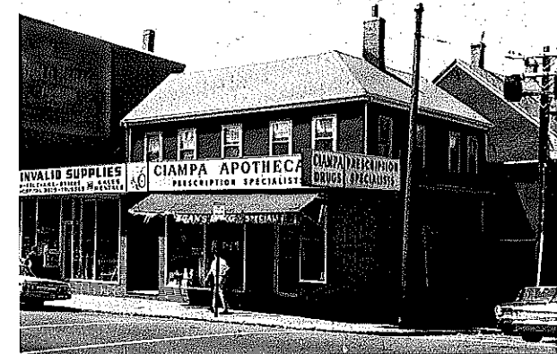
340. 425 Cambridge Street, 1824-25. Photograph 1969
