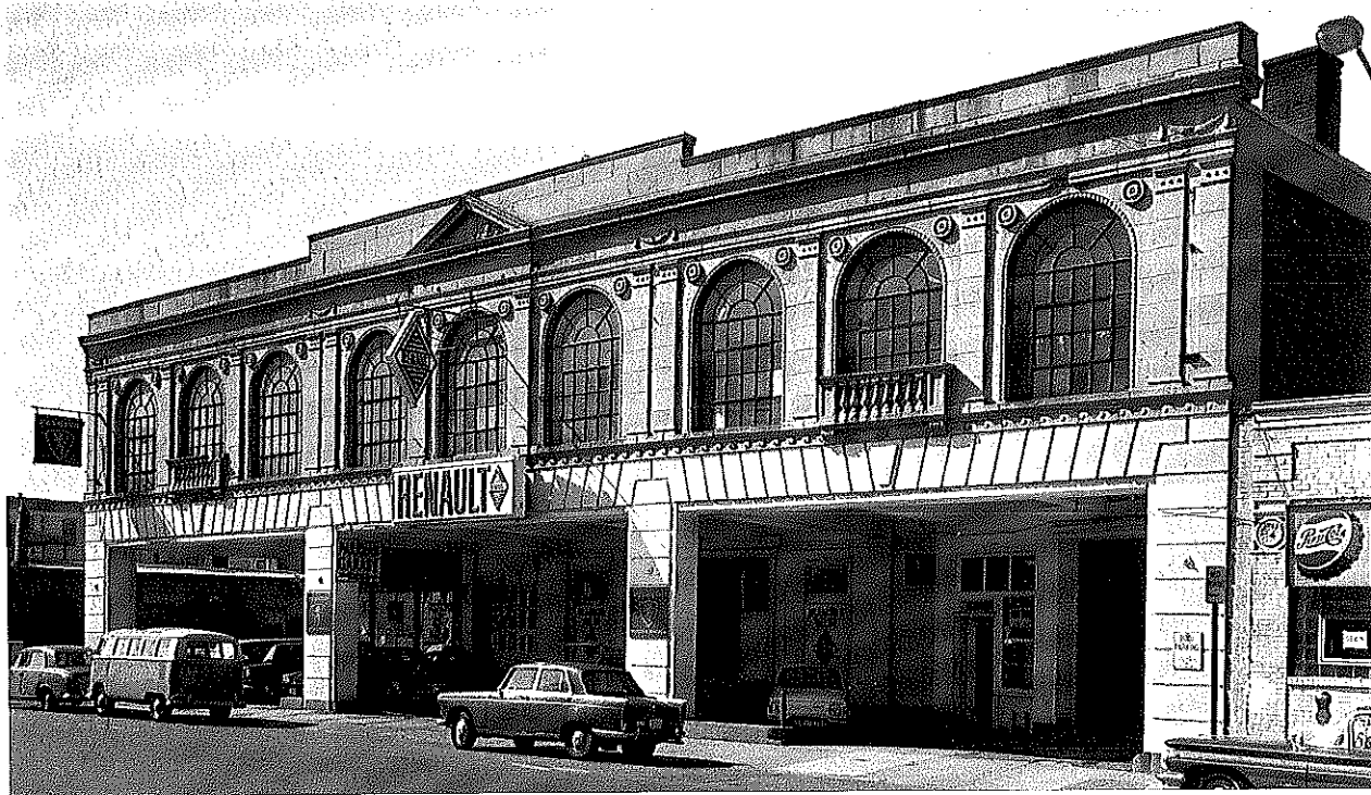
342. East Cambridge Garage, 665 Cambridge Street, 1927, S. S. Ersulag. Demolished 1974. Photograph 1969
