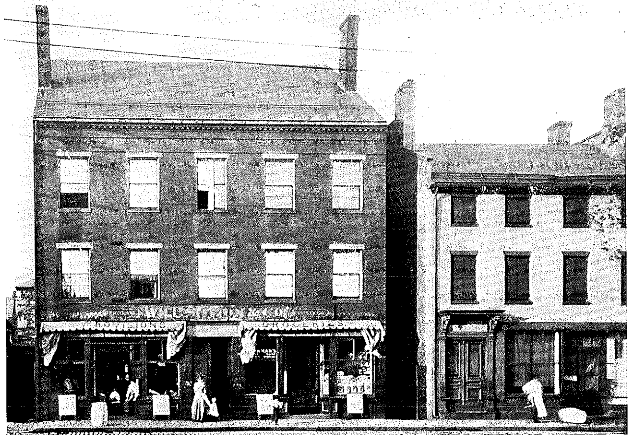
328. Reed's Hall, 161 Bridge Street, c. 1840. Demolished c. 1925. Photograph 1904
