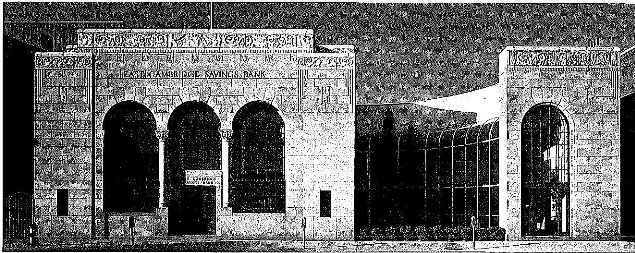
325. East Cambridge Savings Bank, 292 Cambridge Street, 1931, Thomas M. James, Addition (right), 1976, Charles Hilgenhurst Associates
