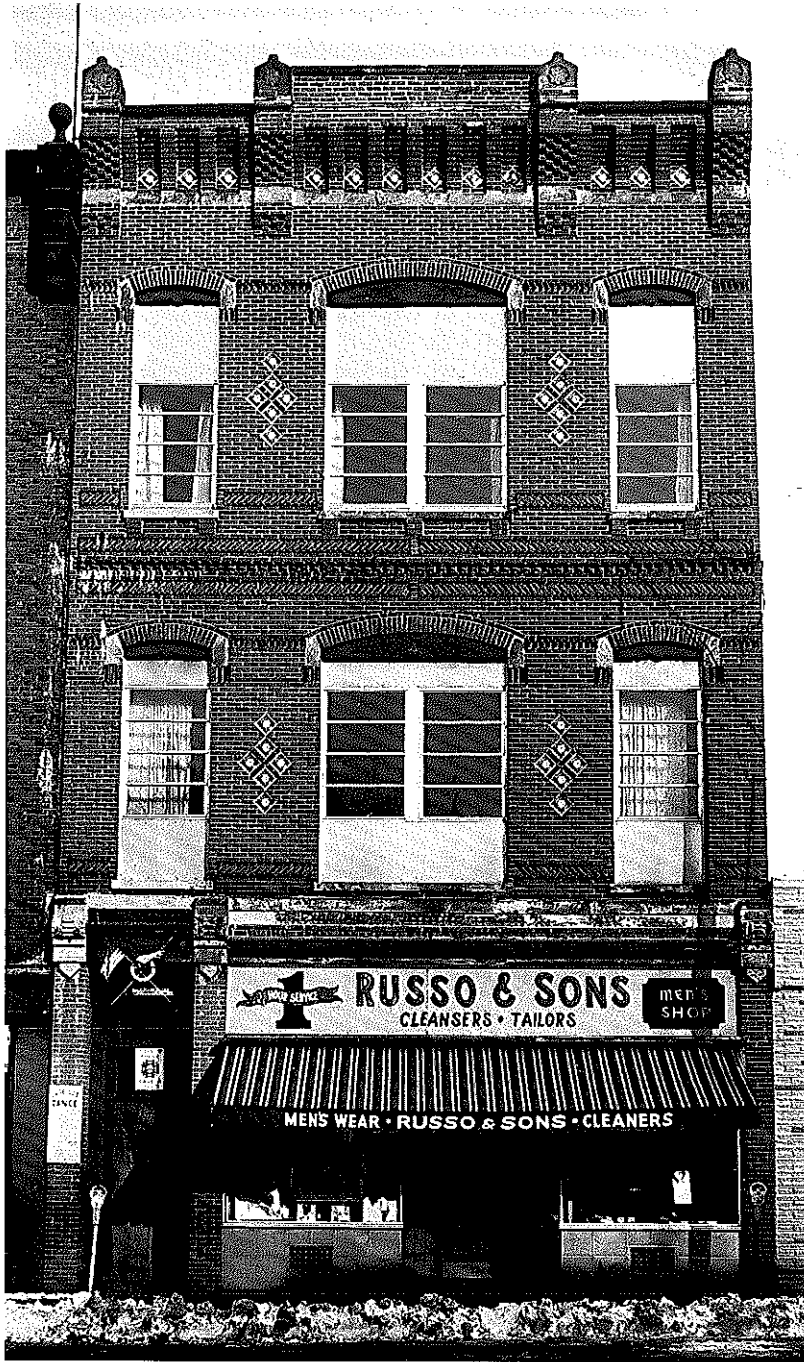
331. 305 Cambridge Street, 1877. Photograph 1964
