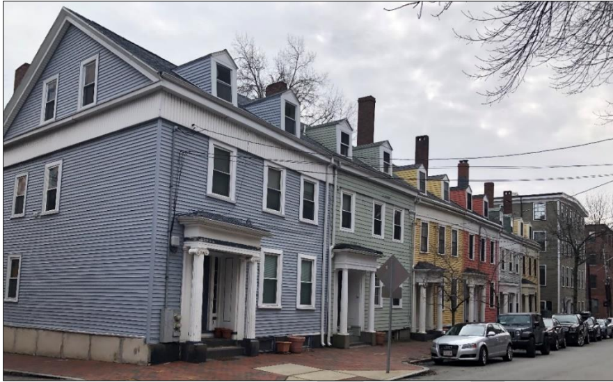
Greek Revival rowhouses (1842) at 36-46 Second Street
