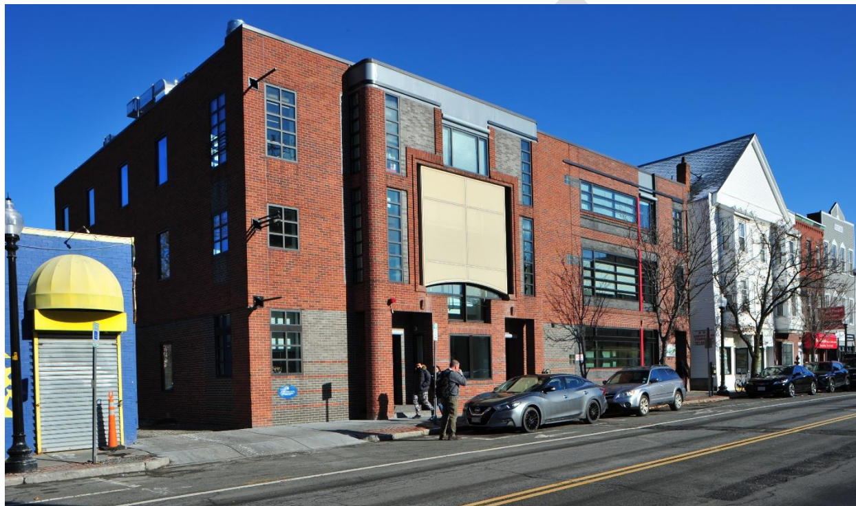
Case 4323: 271 Cambridge Street after renovation.
