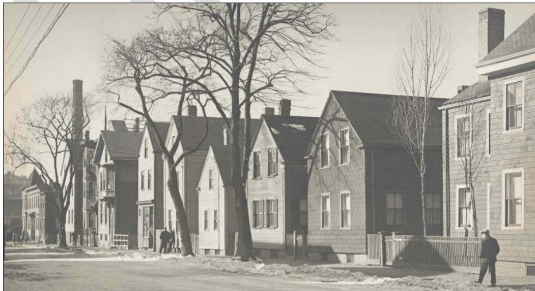
Winter Street Worker's Cottages, c.1940
