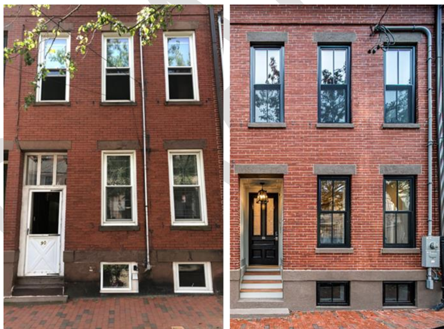
Case 4215: 90 Thorndike Street façade before and after administrative permit review.
