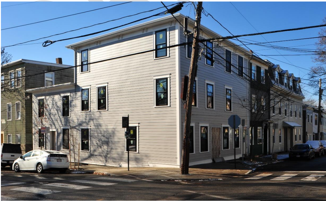
Case 4267: 118 Spring Street after renovation
