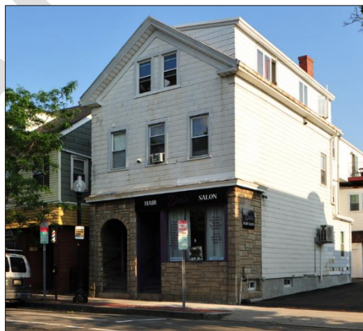
450 Cambridge Street (1856) with inserted storefront from 1901. CHC
