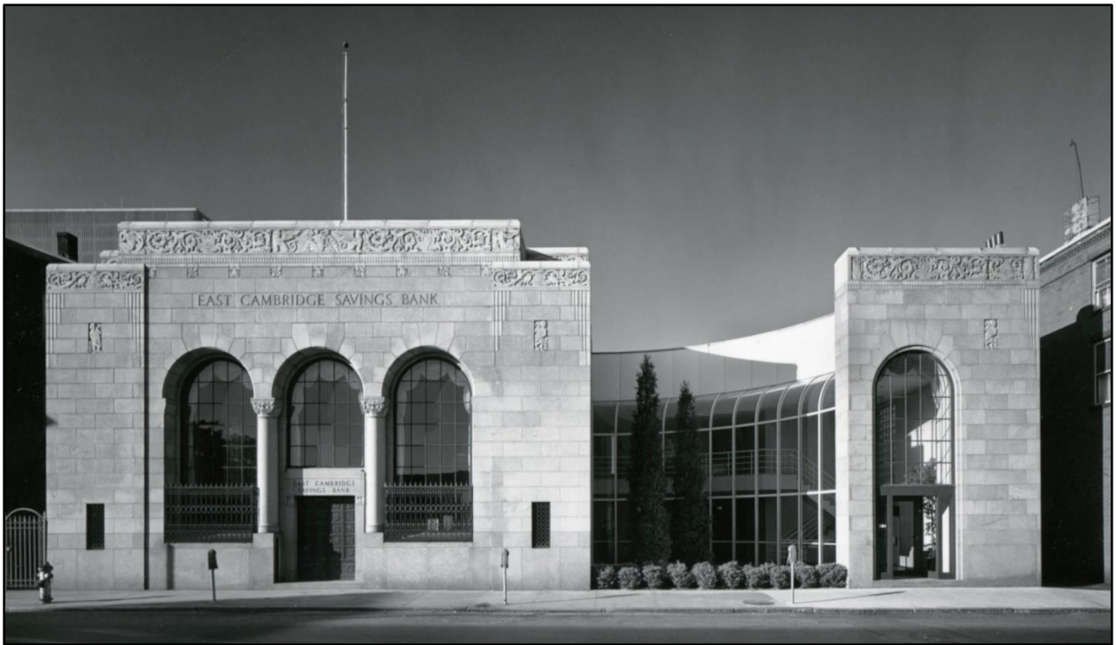
East Cambridge Savings Bank, constructed in 1931 (left), with 1977 addition (right).
