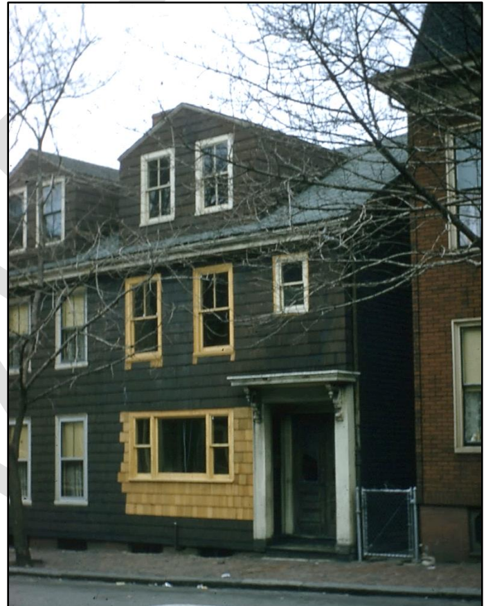
137 Otis Street ca.1946, with recently added picture window.
