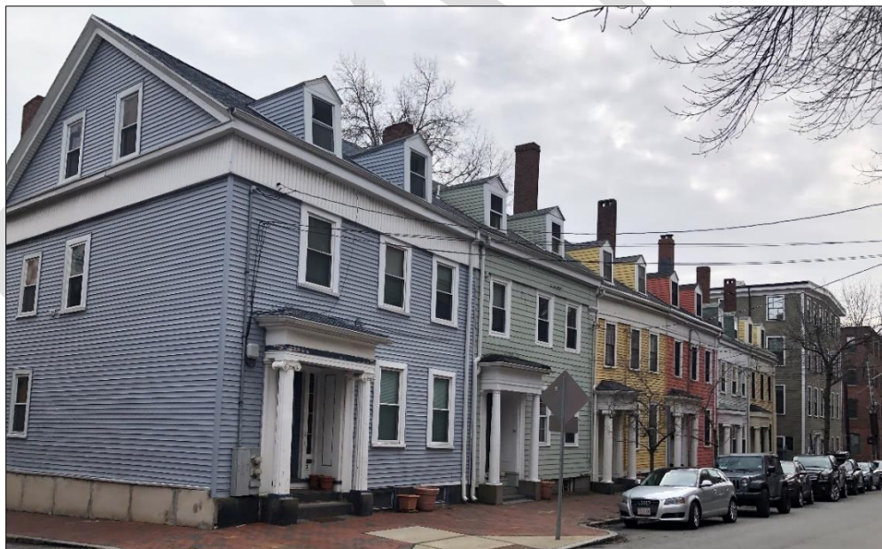
Greek Revival rowhouses (1842) at 36-46 Second Street
