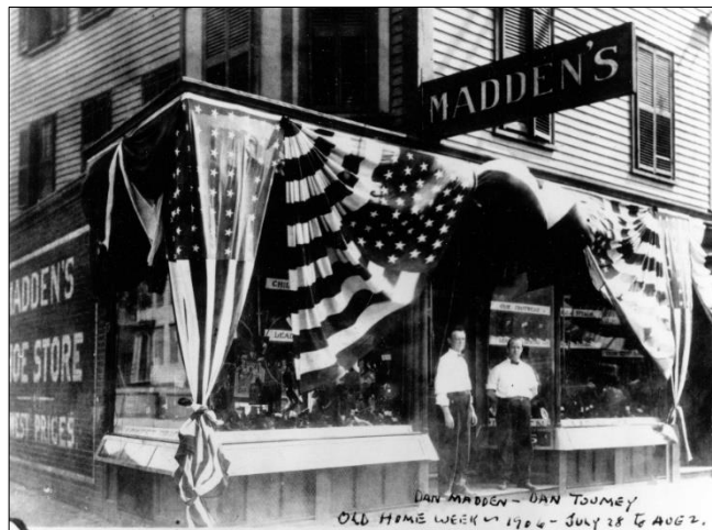
635 Cambridge Street (1867) with new storefront, 1906.
