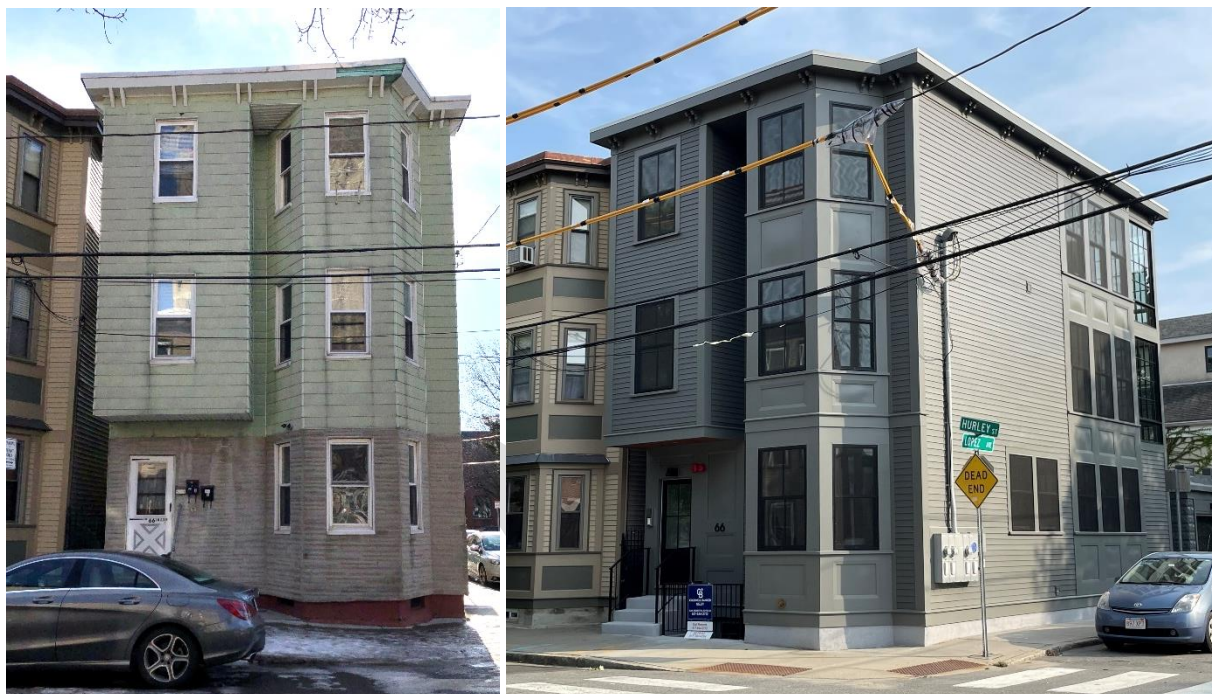
Case 4280, 66 Hurley Street (1907), before and after a renovation project that was granted a Certificate of Appropriateness in 2019. CHC photos, 2019 and 2021
