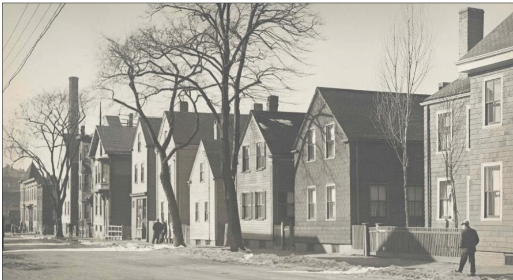
Winter Street Worker's Cottages, c.1940
