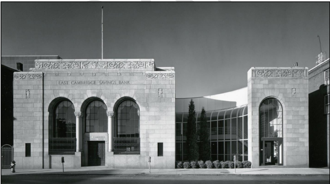
East Cambridge Savings Bank, constructed in 1931 (left), with 1977 addition (right).
