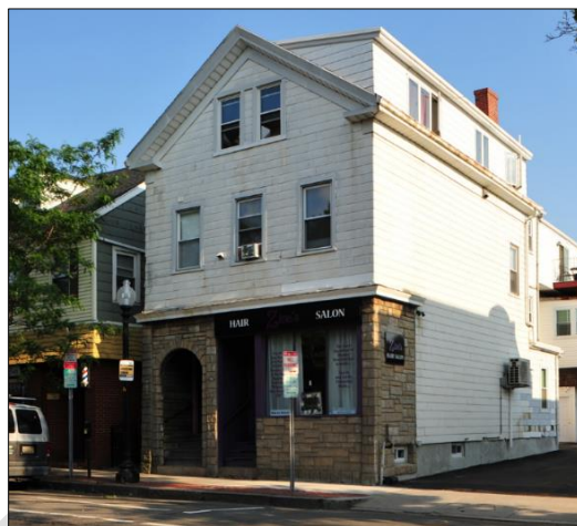
450 Cambridge Street (1856) with inserted storefront from 1901. CHC
