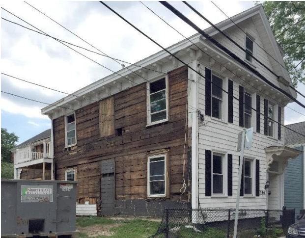
156 Thorndike Street with chimneys, porch and siding removed, showing the original window pattern and cornice brackets. CHC staff photo, June 2017.
