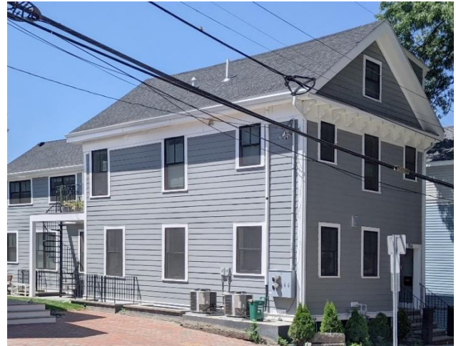
156 Thorndike Street as completed, showing removal of cornice brackets and random placement and sizes of windows. CHC staff photo, July 2022
