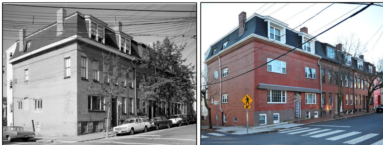
84-94 Thorndike Street in 1970 (left) and 2020 (right). Changed window configuration disrupted the continuity of the block.
