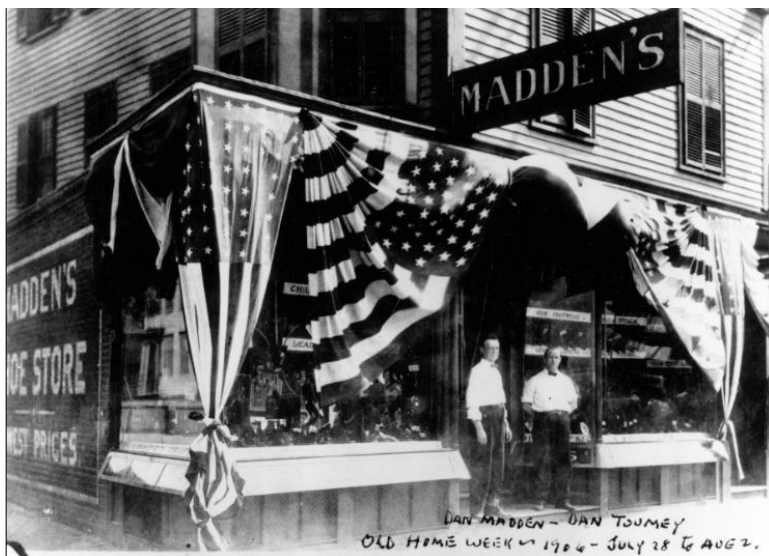
635 Cambridge Street (1867) with new storefront, 1906 CHC
