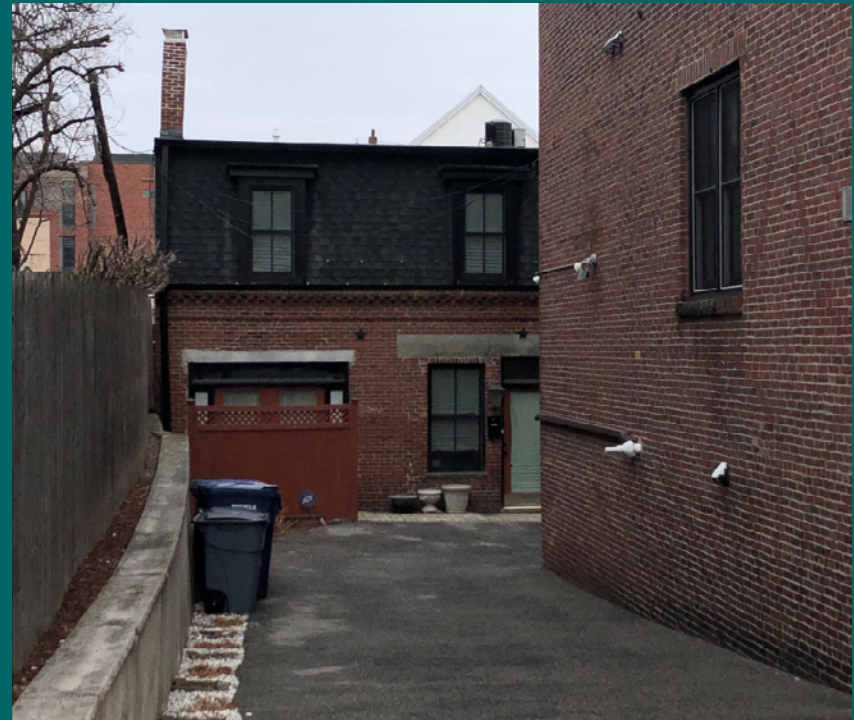
65 Otis Street, 1880s stable converted into two attached units.
