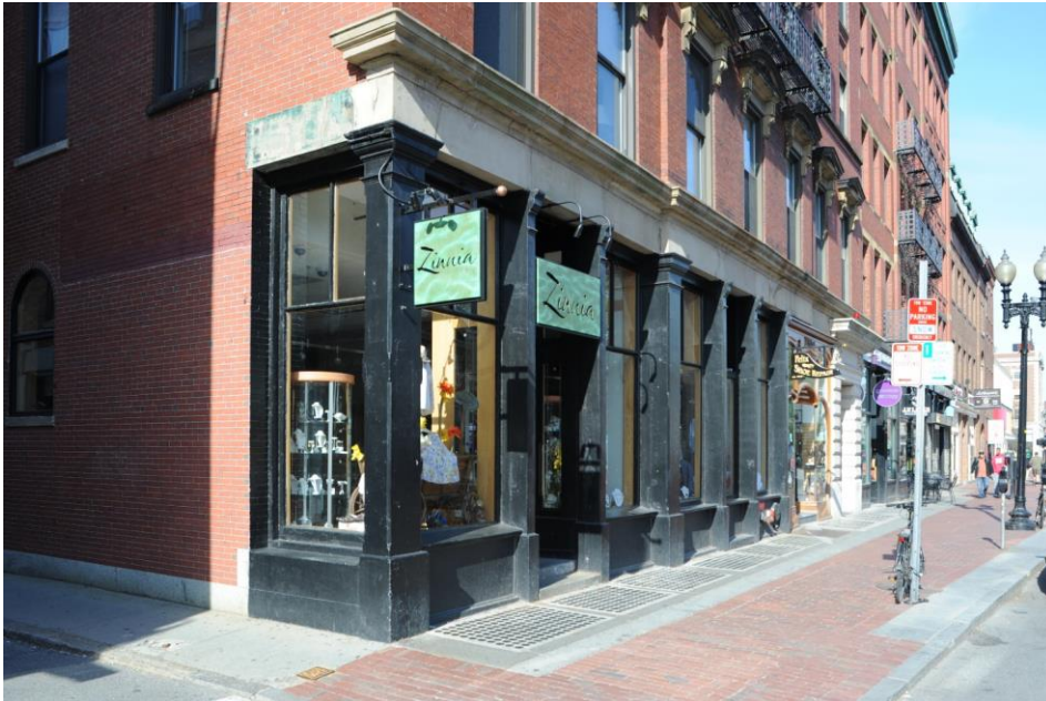
Restored storefronts, 1300-1310 Massachusetts Avenue
