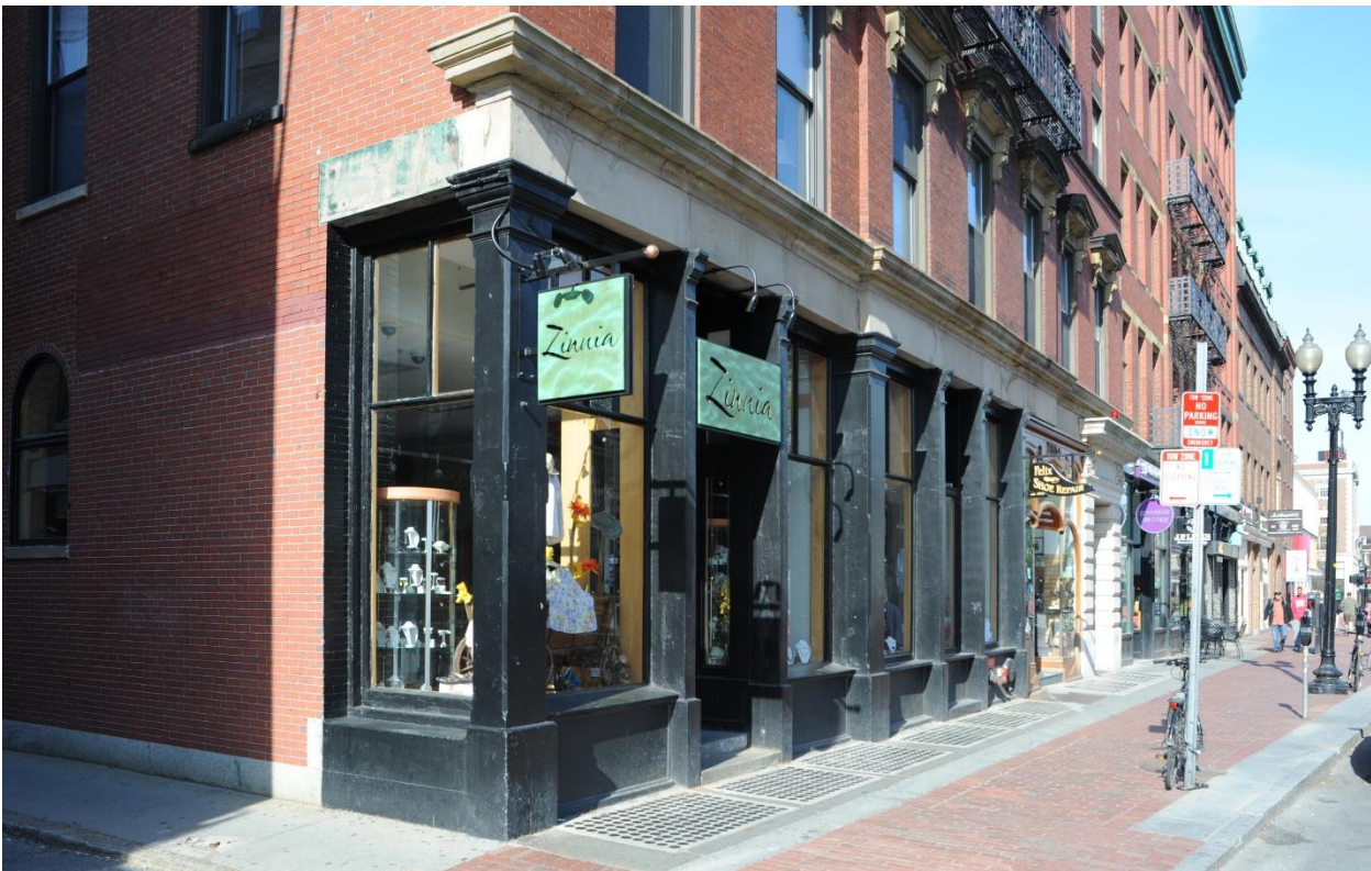
Storefronts restored by removal of later accretions, 1300-1310 Massachusetts Avenue
