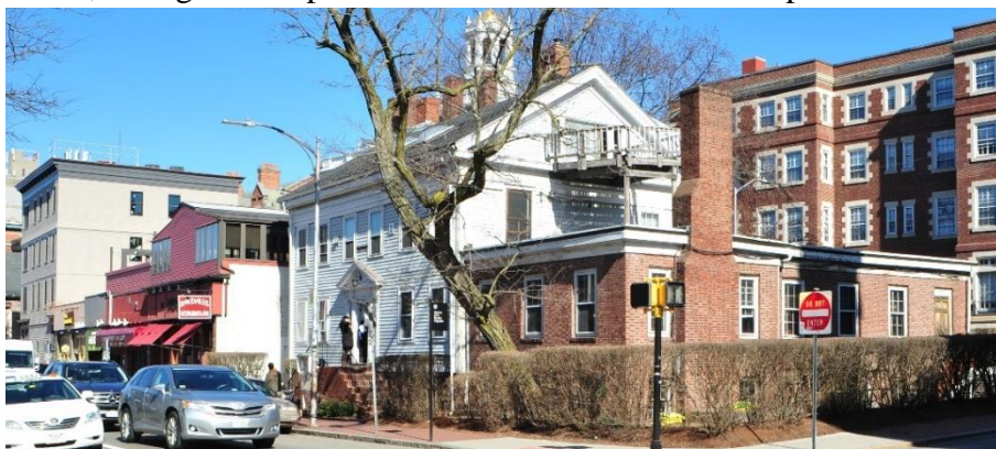
43-45 Mt. Auburn St. (1846, addition 1928). 45-49 Mt. Auburn (1971, 1926) at left
