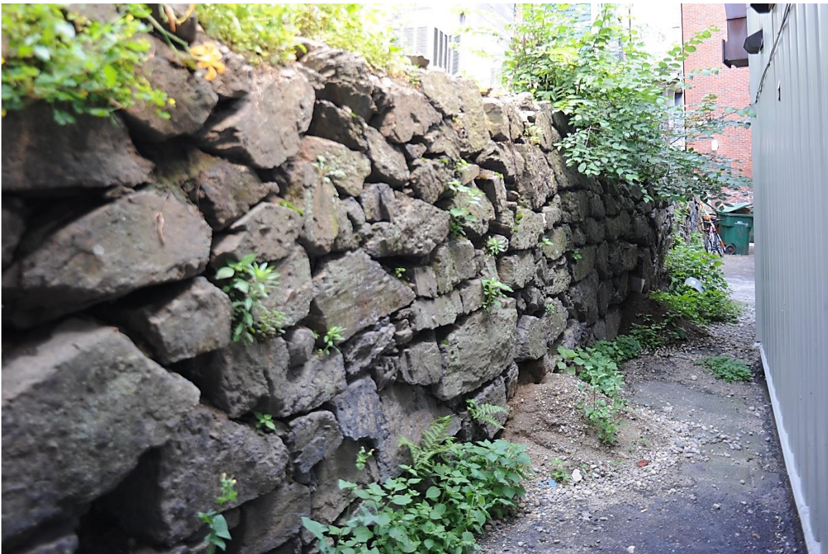
Winthrop Street retaining wall (ca. 1800), behind 16 Eliot Street
