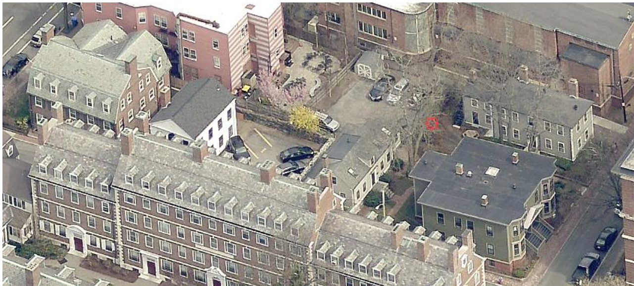
South Street (behind Bryan Hall) and Dunster Street (right), with 60 JFK Street (1929), 21 South Street (1956), 17 South Street (1824), and 71-77 Dunster Street (1894) and 69 Dunster Street (1829). Cambridge GIS, 2014
