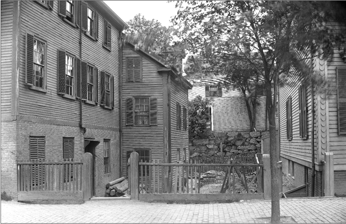
Winthrop Street retaining wall, as seen between 8 and 10-14 Eliot Street, 1909
