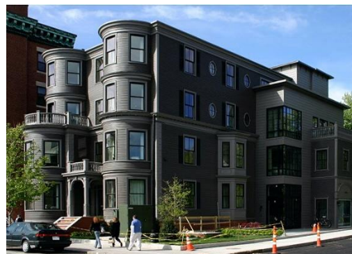
Veritas Hotel, 1131 Massachusetts Avenue
