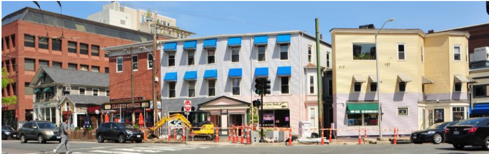
8 Eliot Street (ca. 1790); 8A Eliot (1989, Benjamin Thompson Associates, architects); 10 and 12-14 Eliot (1869); and 14A Eliot (1900).
