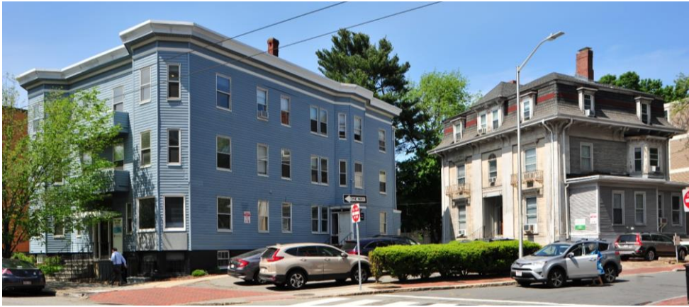
127 Mt. Auburn Street (1912) and the Munroe-Jacobs Jacobs house, 17 Story Street (1846).
