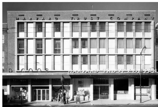
Harvard Trust Co. façade, 1408-1414 Massachusetts Ave. Photo ca. 1958.
