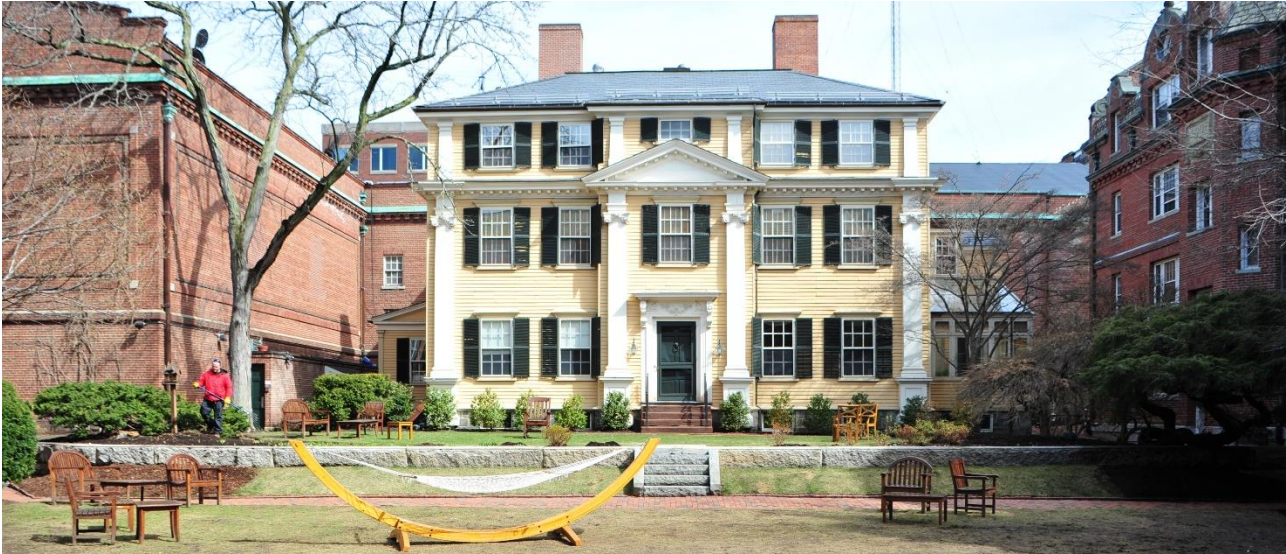
Aphthorp House (1760), in the Randolph Hall courtyard.
