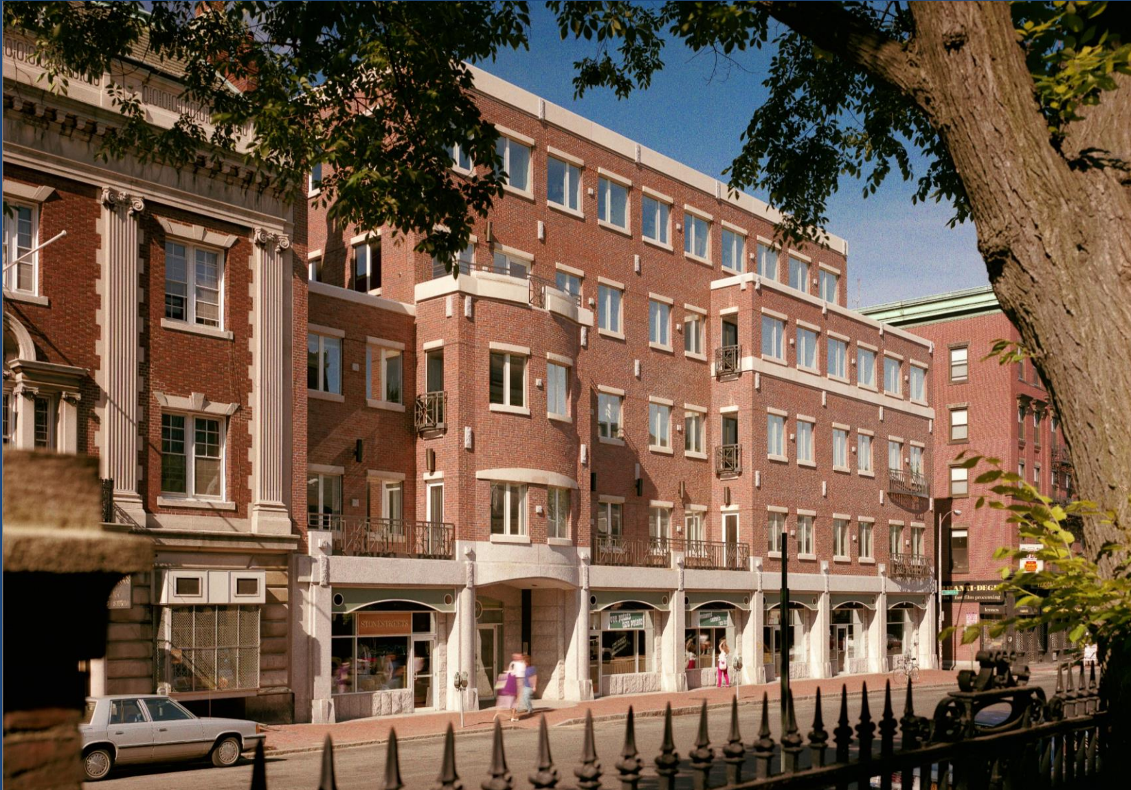
Niles Building, 1280 Massachusetts Avenue (1983, Symmes Maini & McKee Associates, architects). Photo 1986
