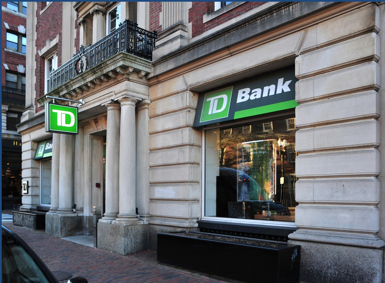
Case 1497: 1270 Mass. Ave. Storefront changes within masonry surround (March 2004)
