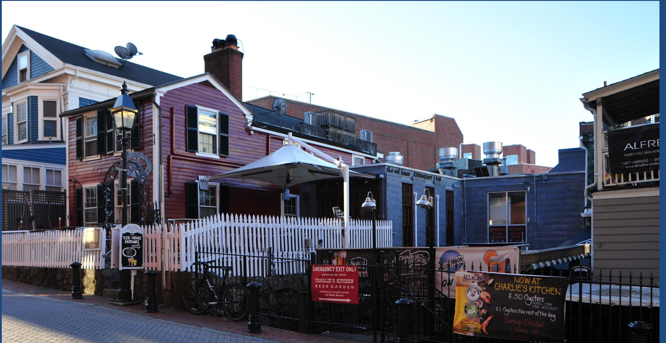
Case 1138: 98 Winthrop Street. Additions and bridge to 10 Eliot Street (August 2001)
