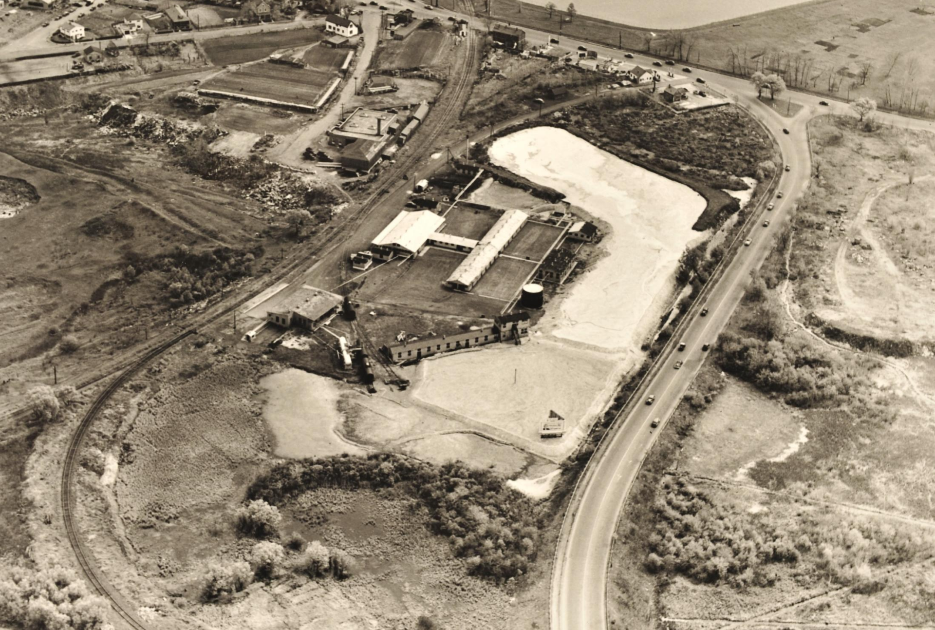
Pres-to-Lite acetylene plant, Alewife Brook Parkway near Concord Avenue, 1948
