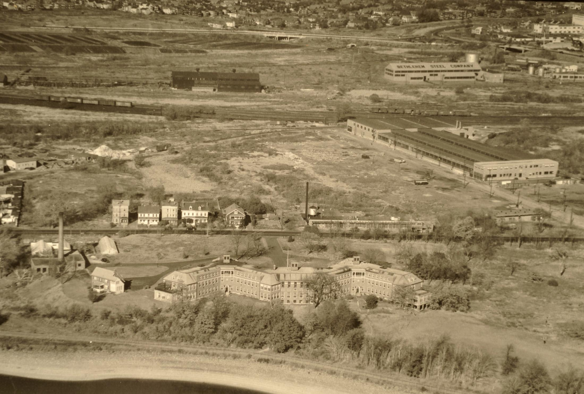
Looking North over Neville Manor, ca. 1950
