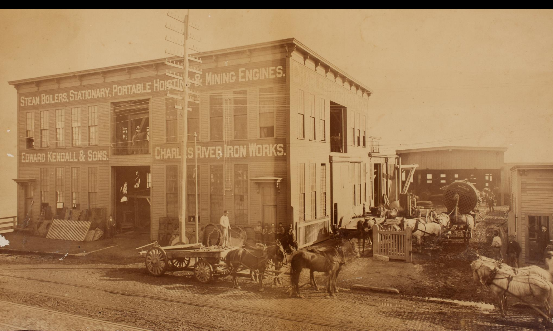
Edward Kendall & Sons, 134 Main Street (site of E62)
