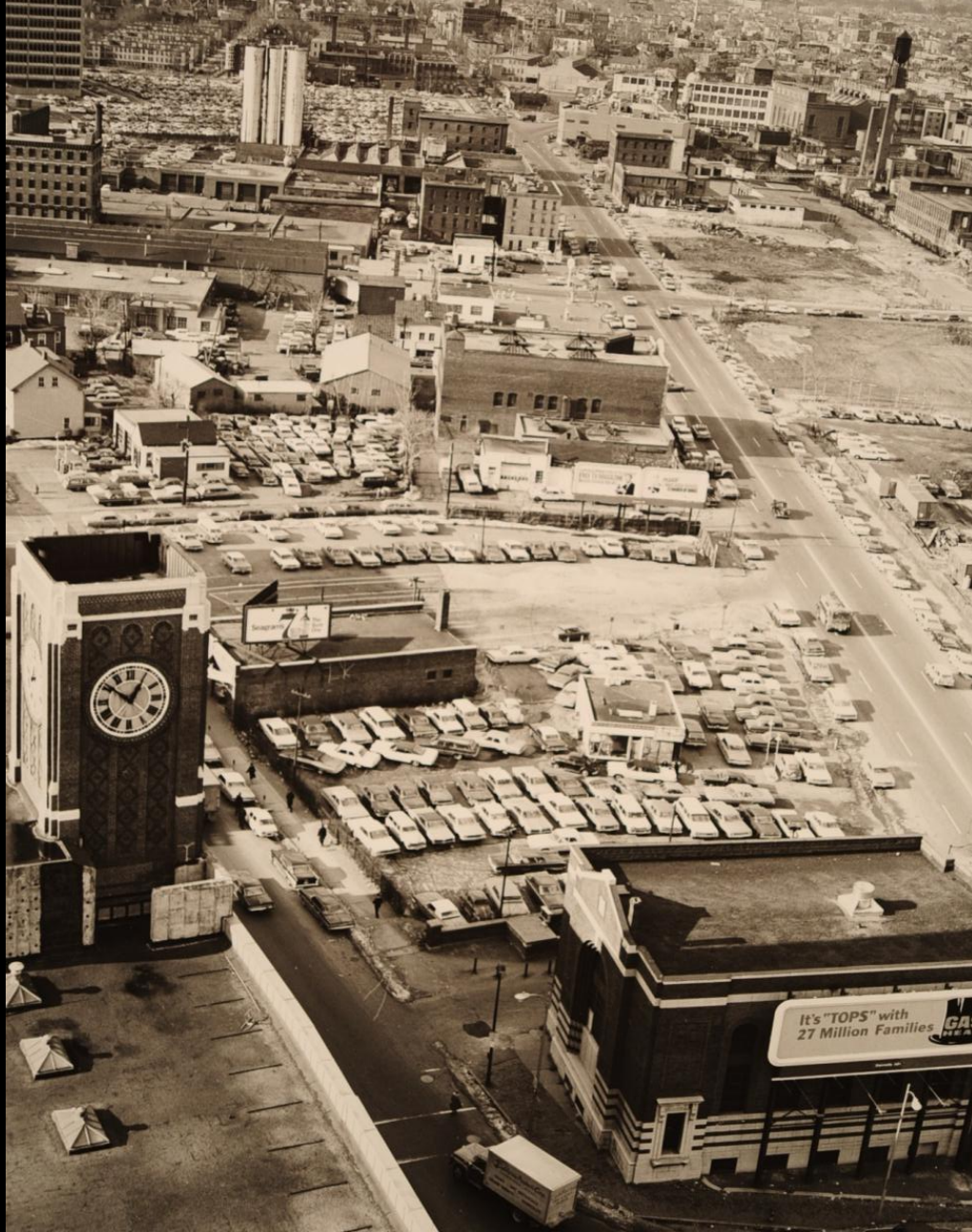
Kendall Square with clearance underway, 1975
