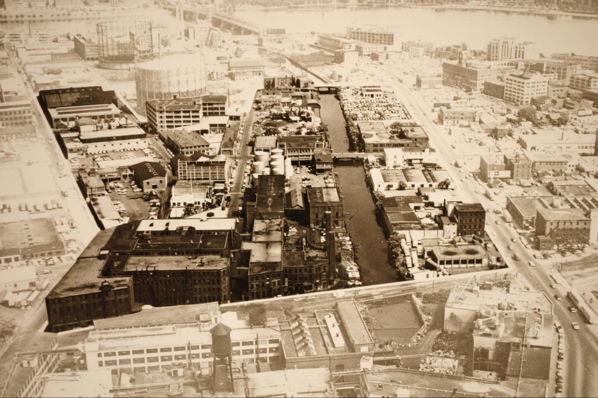
Kendall Square Urban Renewal Project Area, 1960
