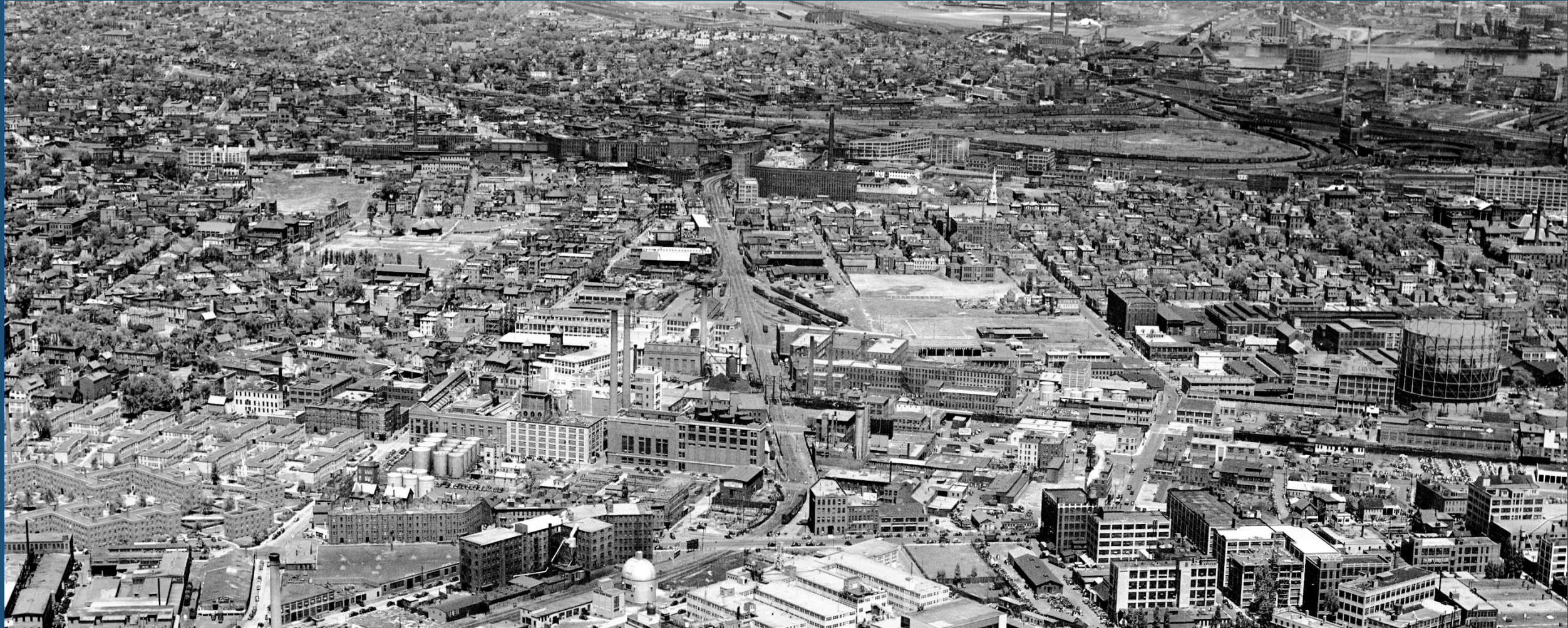
Industrial Corridor between East Cambridge and Donnelly Field, 1957
