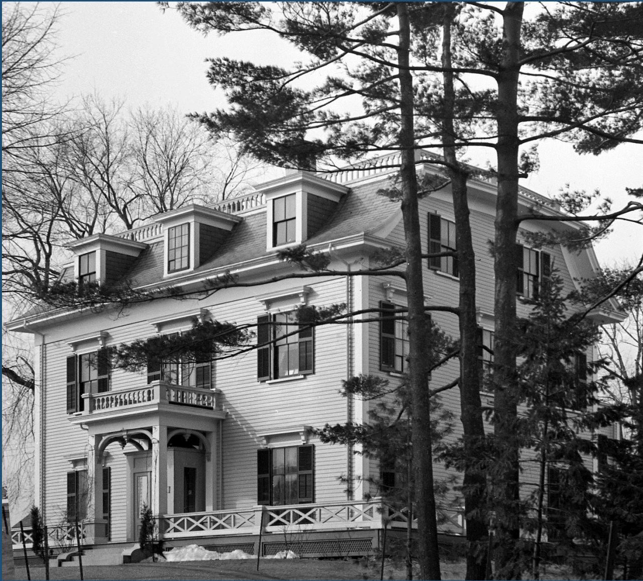
Dr. Morrill Wyman house, 77 Sparks Street (1860; demolished 1945). Current site of Hemlock Road. Photo ca. 1938.
