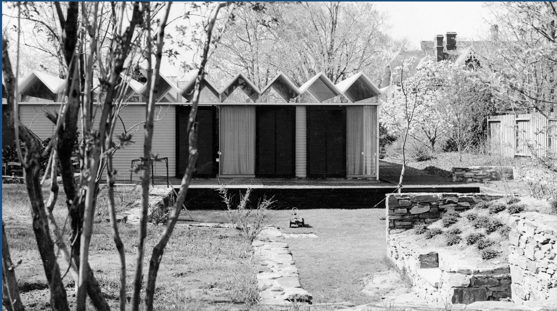
William Wainwright house, 61 Highland Street (1958, Geometrics, Inc., architect). This view shows the foundation of the Alvin Sortwell house, which remained as a landscape feature after the site was cleared in 2003. Photo ca. 1960.
