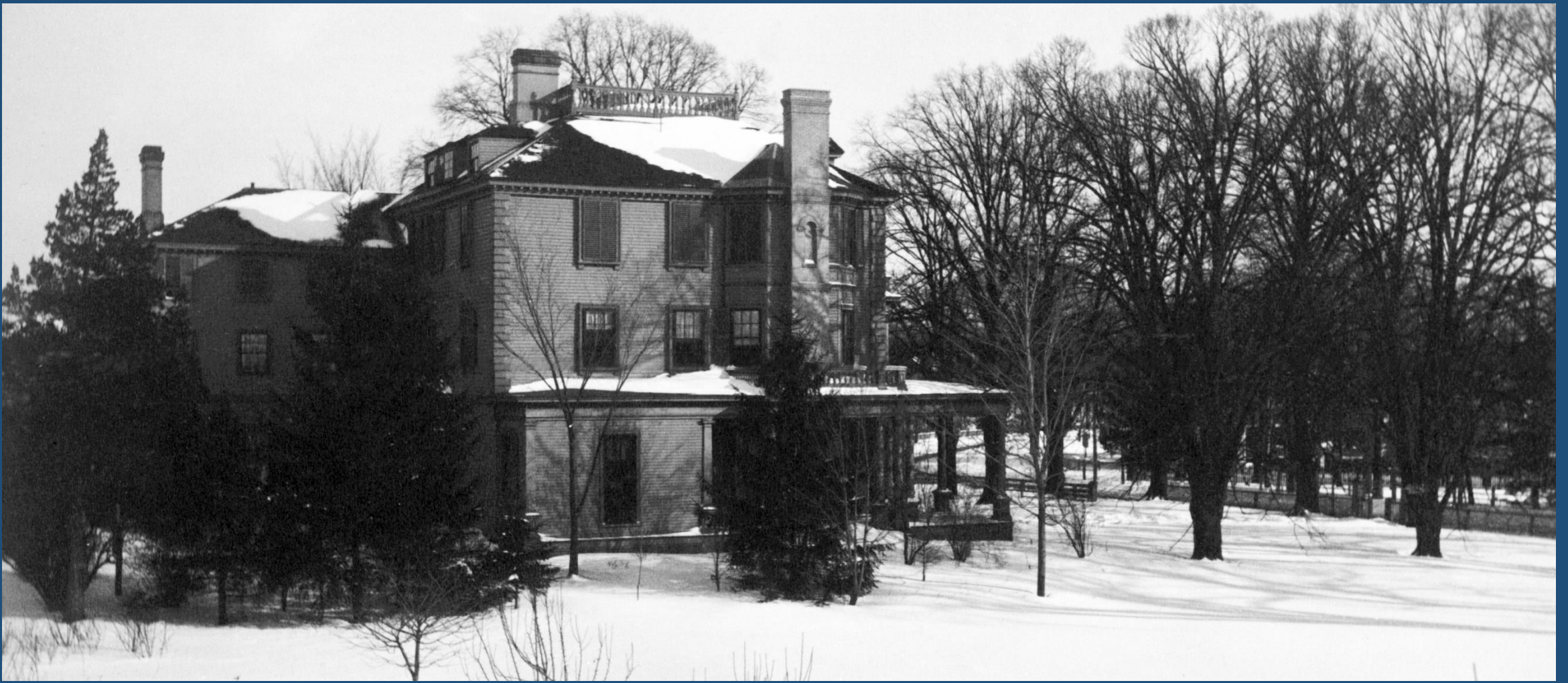
Lechmere-Sewall-Riedesel house on its original site, after John Brewster raised it and inserted a new ground floor in 1869. In 1886 William Brewster removed the original top story and moved the house to 149 Brattle. Photo 1885.
